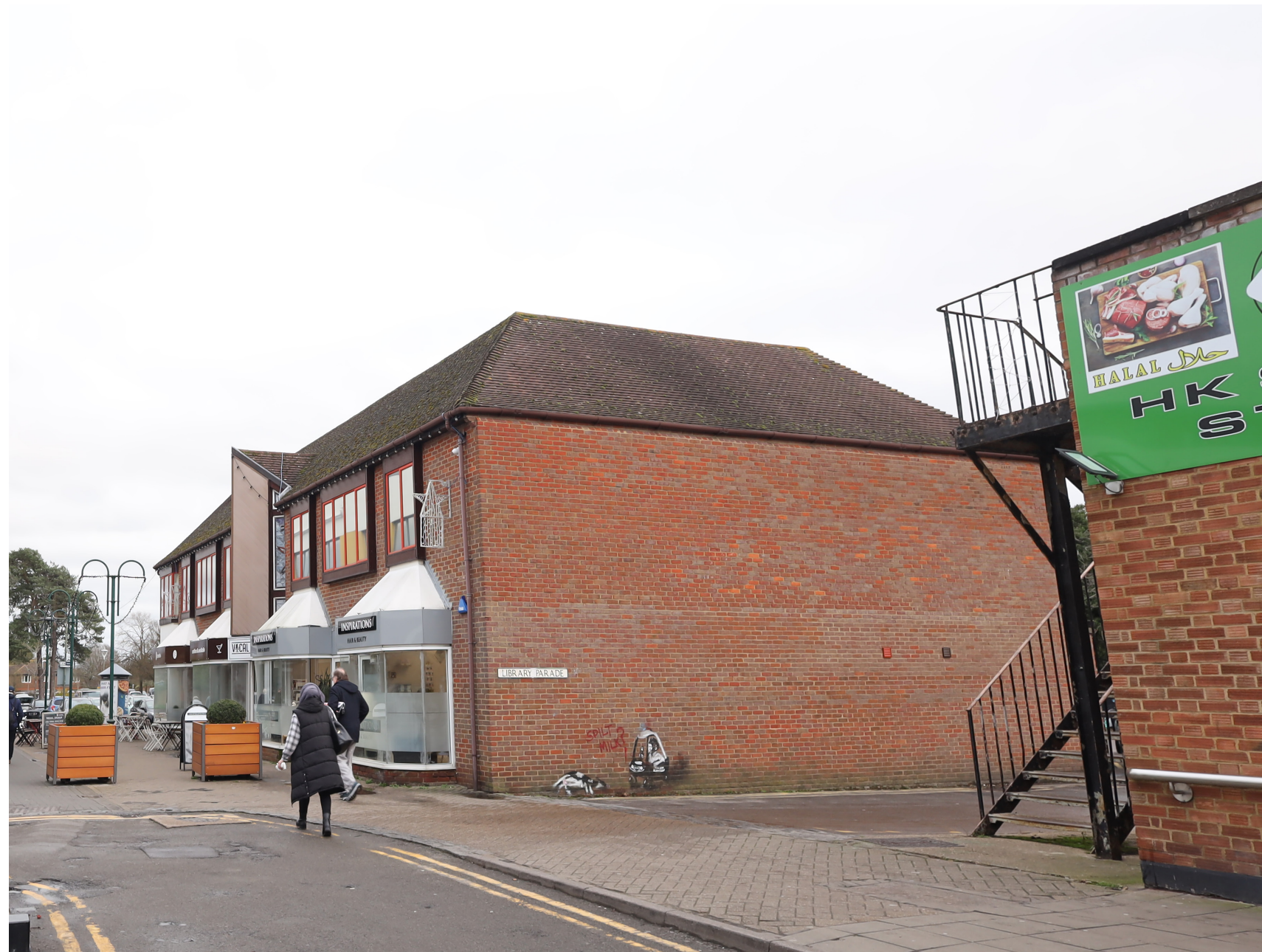
Existing view looking east through Library Parade
