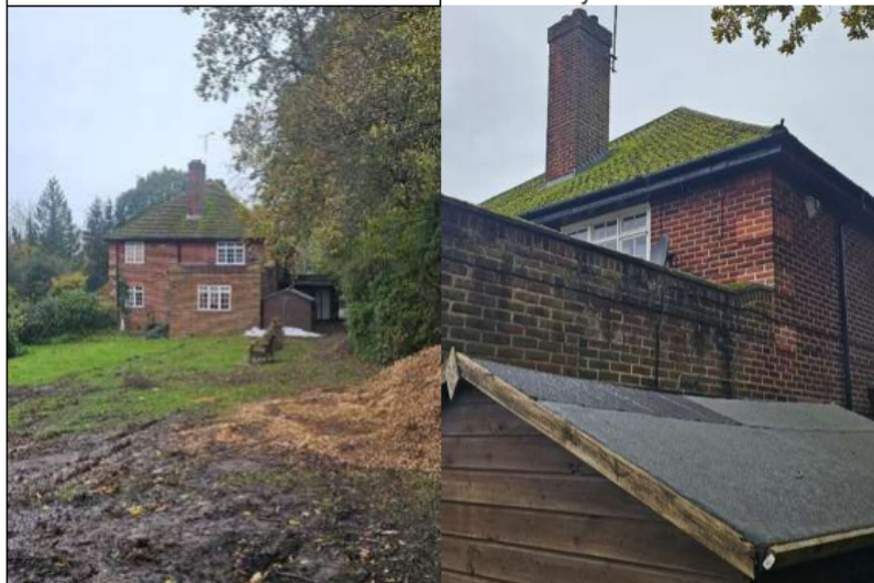
TN 3: Rear elevation of house.
