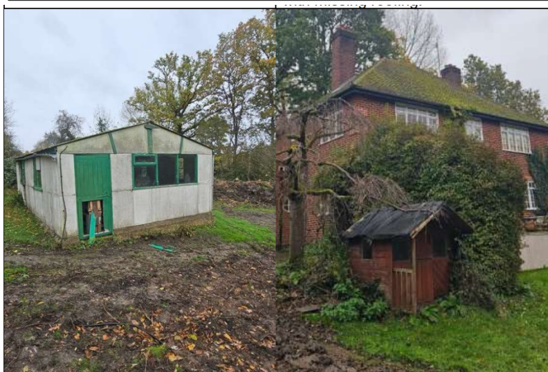
TN 15: Wooden outbuilding.
