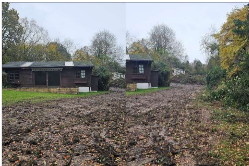
TN 1: Timber clad shed.
