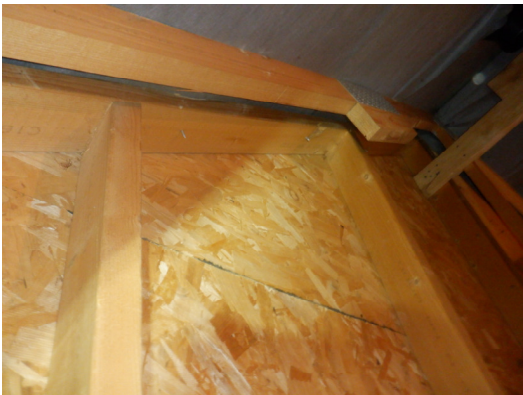
Photograph 13. Southern gable of chipboard construction tight to rafters (roof void).
