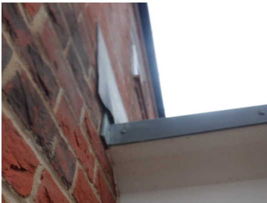
Photograph 5. Lead flashing flush to wall above porch roof (front elevation).
