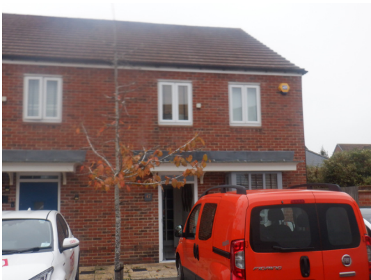
Photograph 1. Front of the property viewed from the west.
