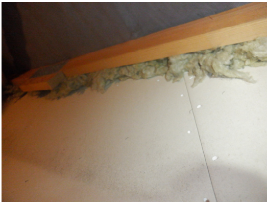
Photograph 12. Fibreglass insulation present around party wall (roof void).
