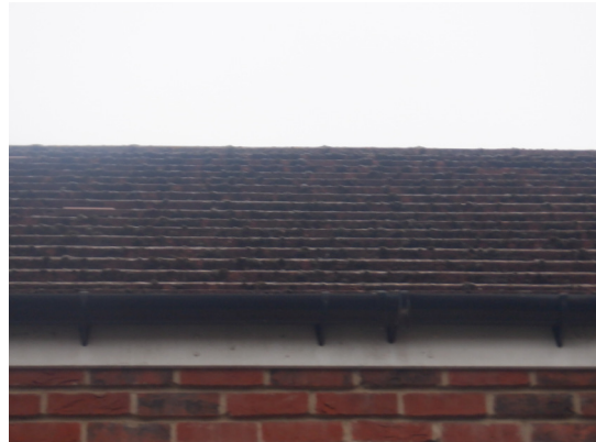
Photograph 4. Tight and intact ridge tiles (front elevation).
