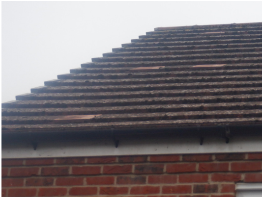
Photograph 3. Flat roof tiles with vents (rear elevation).
