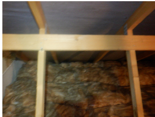
Photograph 11. Fibreglass insulation on floor filling the eaves (roof void).
