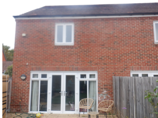
Photograph 2. Rear of the property viewed from the east.
