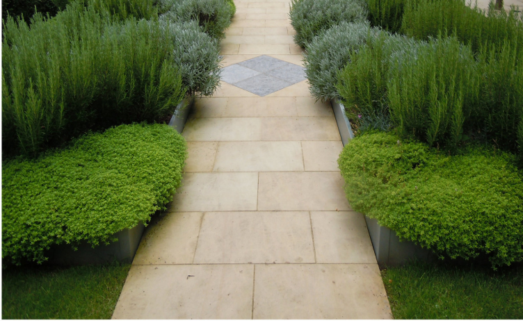
(2) Stone Flags on Terraces - Yorkshire paving slabs
