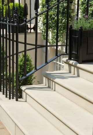
(4) Stone Steps with Metal Balustrading
