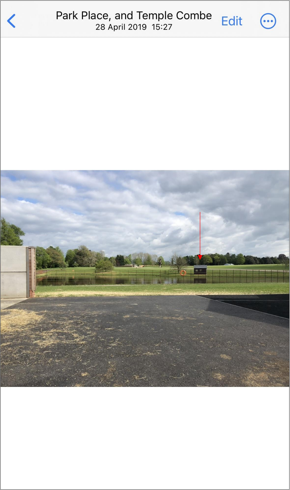
Fig. 8 – Photograph taken by Polo Manager ( ) showing the completed pump house building in situ
