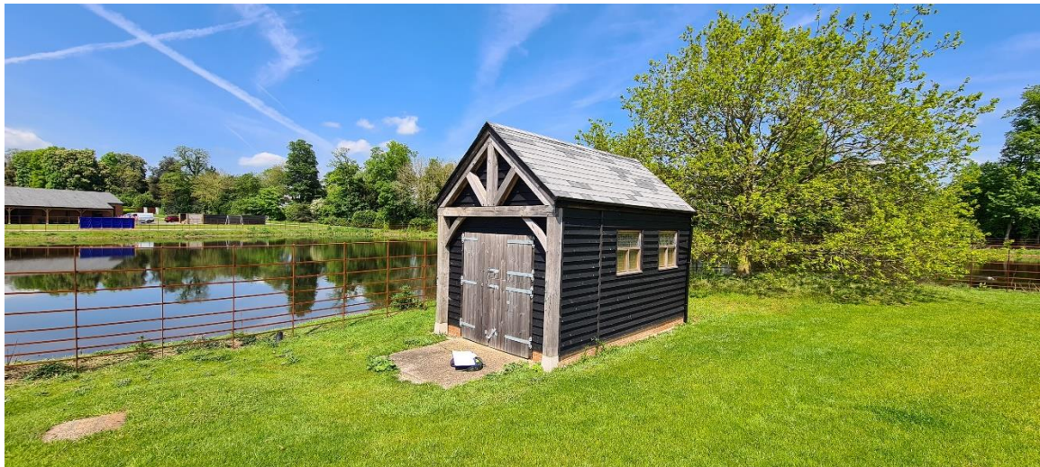
Fig. 1 – Pump house building (May 2024)
