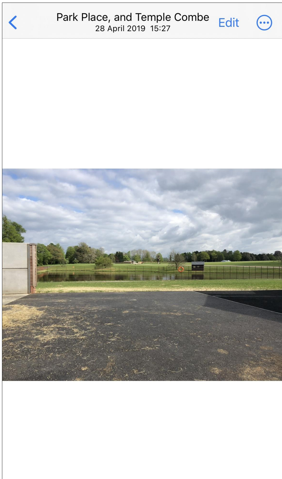
Photo. 1 – Shows the pump house building completed and in situ
