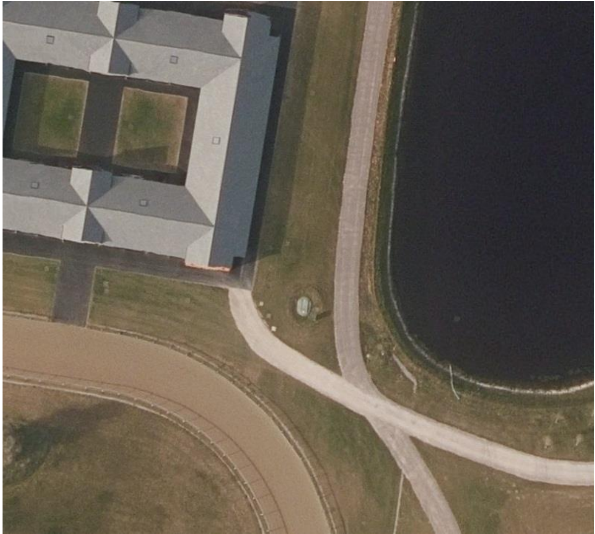
Fig 8. – Date verified aerial photograph (05/04/2020) showing the treatment plant and power unit in situ
