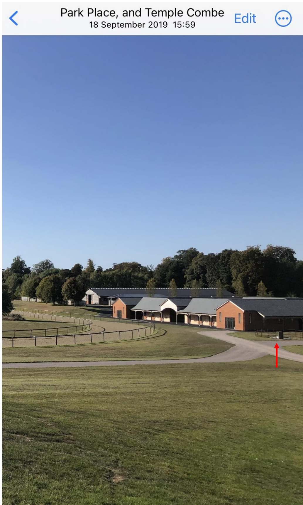
Photo. 1 – Shows the STP and power unit (enclosed by estate fencing)
