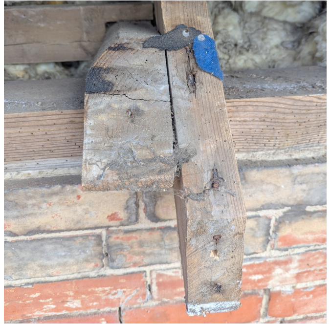
B) Wood worm flight holes
