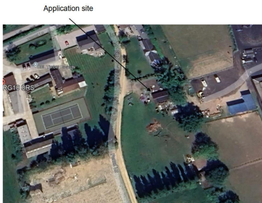
Figure 8: 2025 Aerial Image showing the outbuilding in situ provided by the applicant
