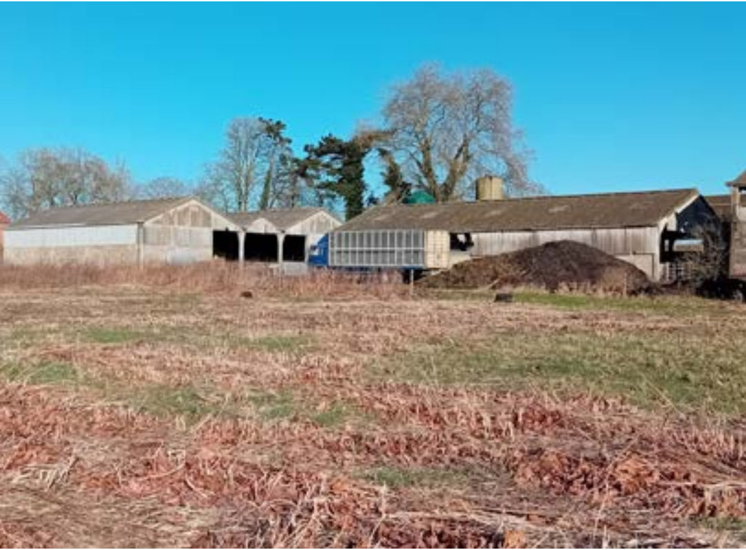
Image of the site looking east from the river bank (Jan 2024)
