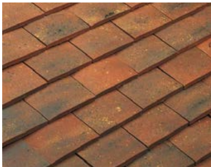
Roof - Orange Clay Tile
