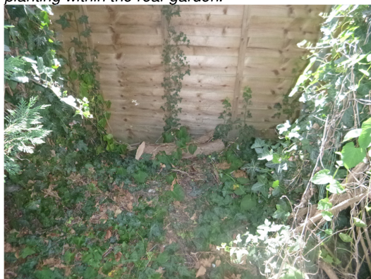
Photograph 7. Timber fence sealed to the ground within the rear garden.
