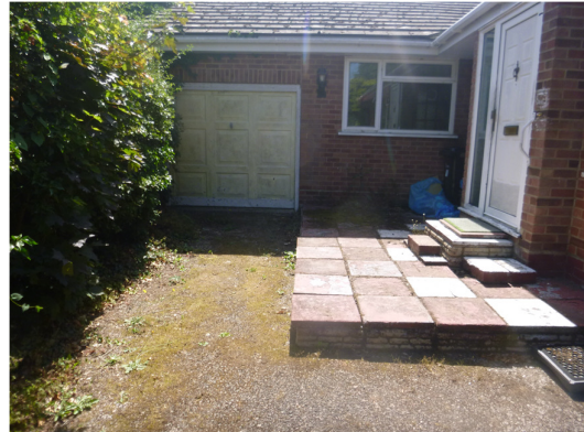
Photograph 2. Patio and hard standing across the front elevation of the property.
