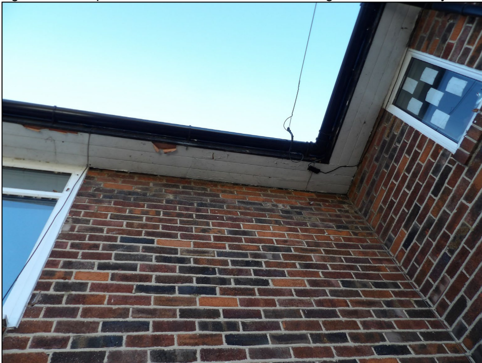
Figure 6. Example sealed soffits/fascias. 628 Wokingham Road, Earley. 26.11.24
