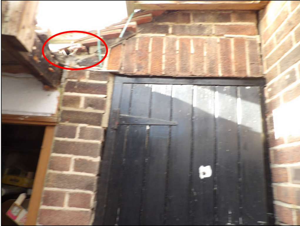
Figure 9. Missing mortar in verge of lean-to section of the property. 628 Wokingham Road, Earley. 26.11.24
