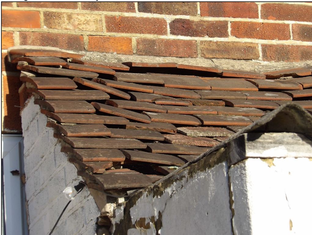
Figure 8. Gaps in tiles covering rear, lean-to style section of the property. 628 Wokingham Road, Earley. 26.11.24
