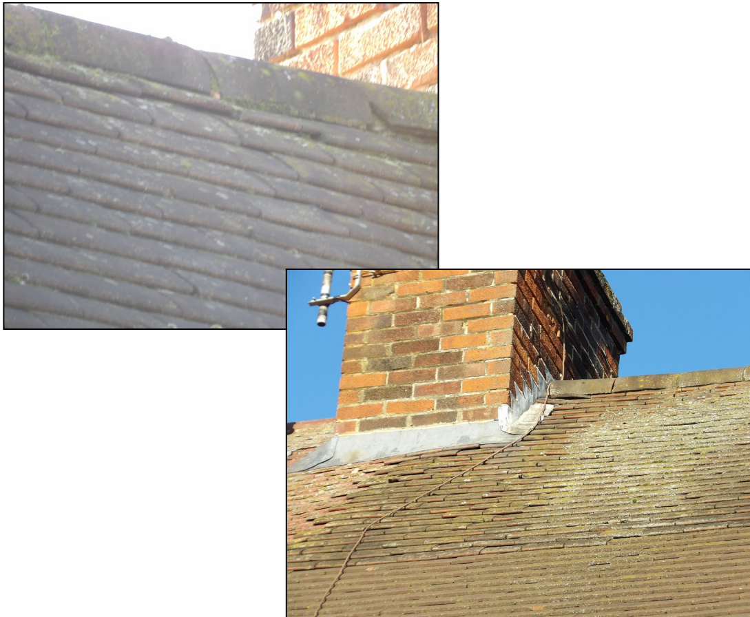
Figure 4. Example moved/raised roof tiles. 628 Wokingham Road, Earley. 26.11.24
