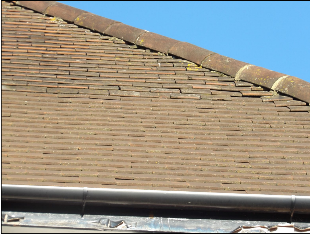
Figure 5. Example missing mortar from hip tiles. 628 Wokingham Road, Earley. 26.11.24
