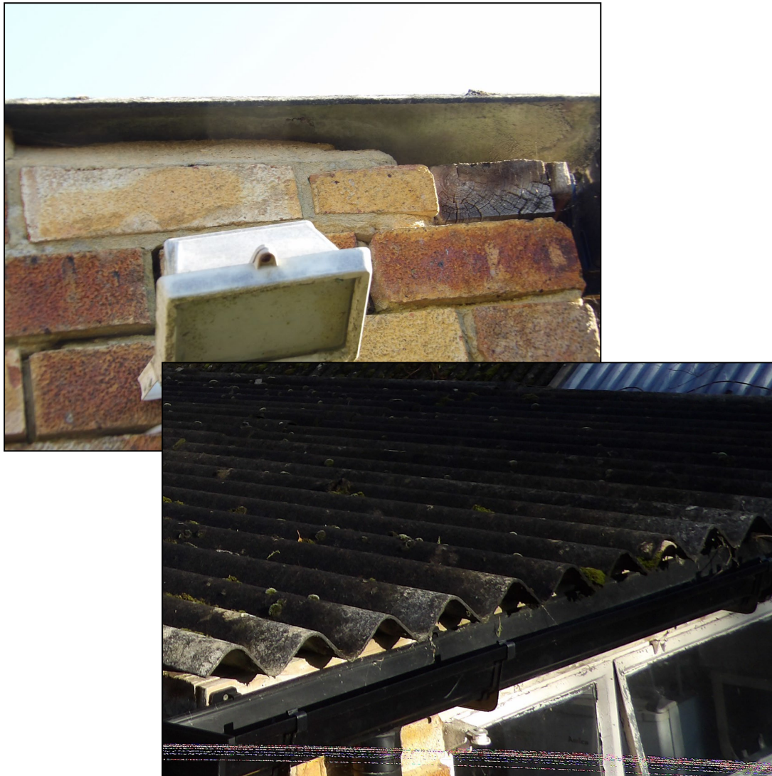
Figure 12. Missing cement/gaps at rear of outbuilding. 628 Wokingham Road, Earley. 26.11.24
