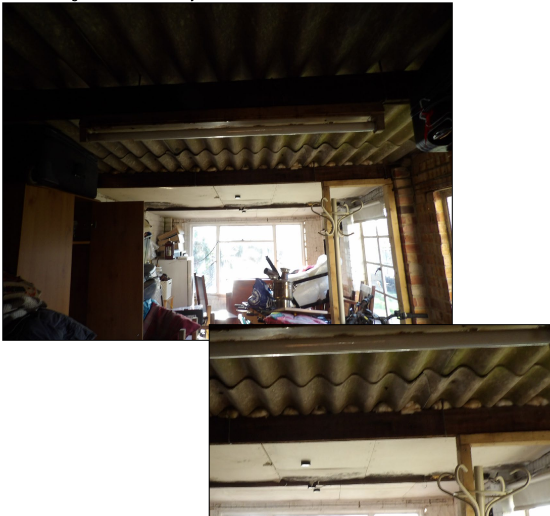
Figure 15. Internal view of outbuilding showing partly lined ceiling and expanding foam. 628 Wokingham Road, Earley. 26.11.24
