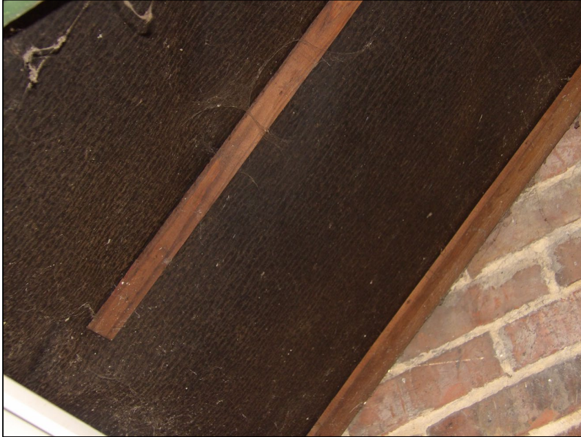
Figure 14. Example of bitumen lining to 'lean-to' building. 628 Wokingham Road, Earley. 26.11.24
