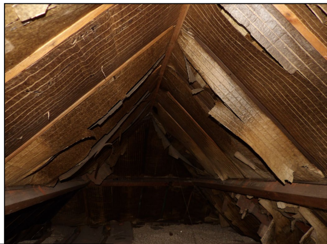
Figure 13. Example loft space and torn tar paper in loft. 628 Wokingham Road, Earley. 26.11.24
