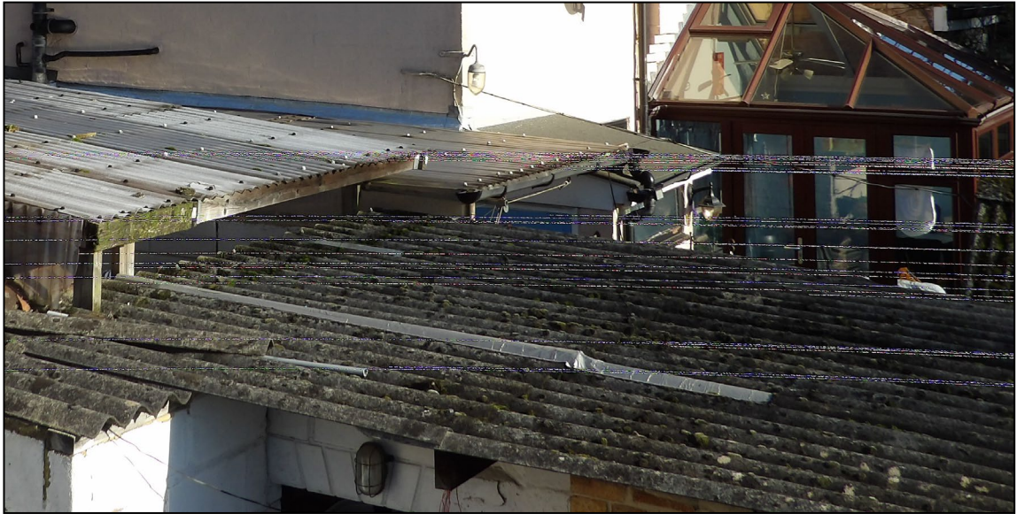
Figure 12. Missing cement/gaps at rear of outbuilding. 628 Wokingham Road, Earley. 26.11.24
