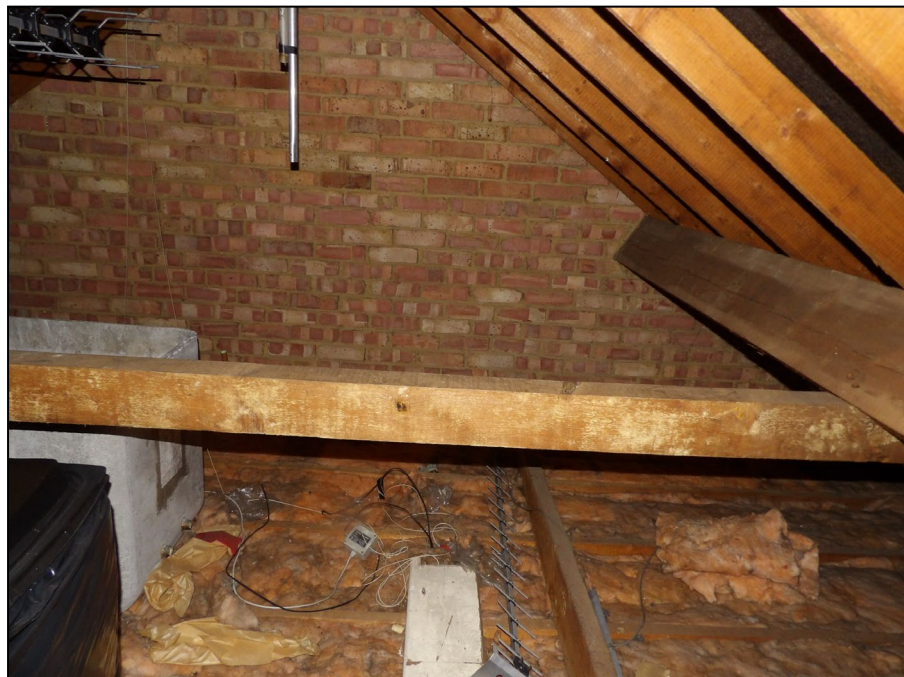
Figure 11. Example of loft space and bitumen lining. 91 London Road, Twyford. 15.07.25
