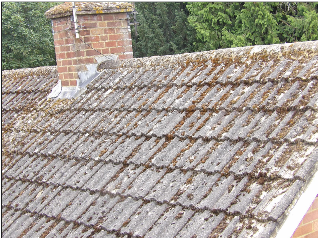
Figure 4. Example of sealed roof/ridge tiles. 91 London Road, Twyford. 15.07.25
