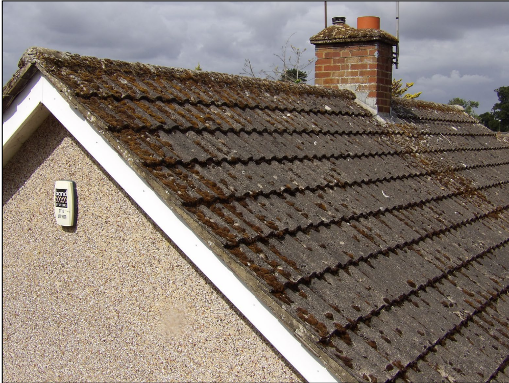
Figure 5. Example of sealed verges. 91 London Road, Twyford. 15.07.25
