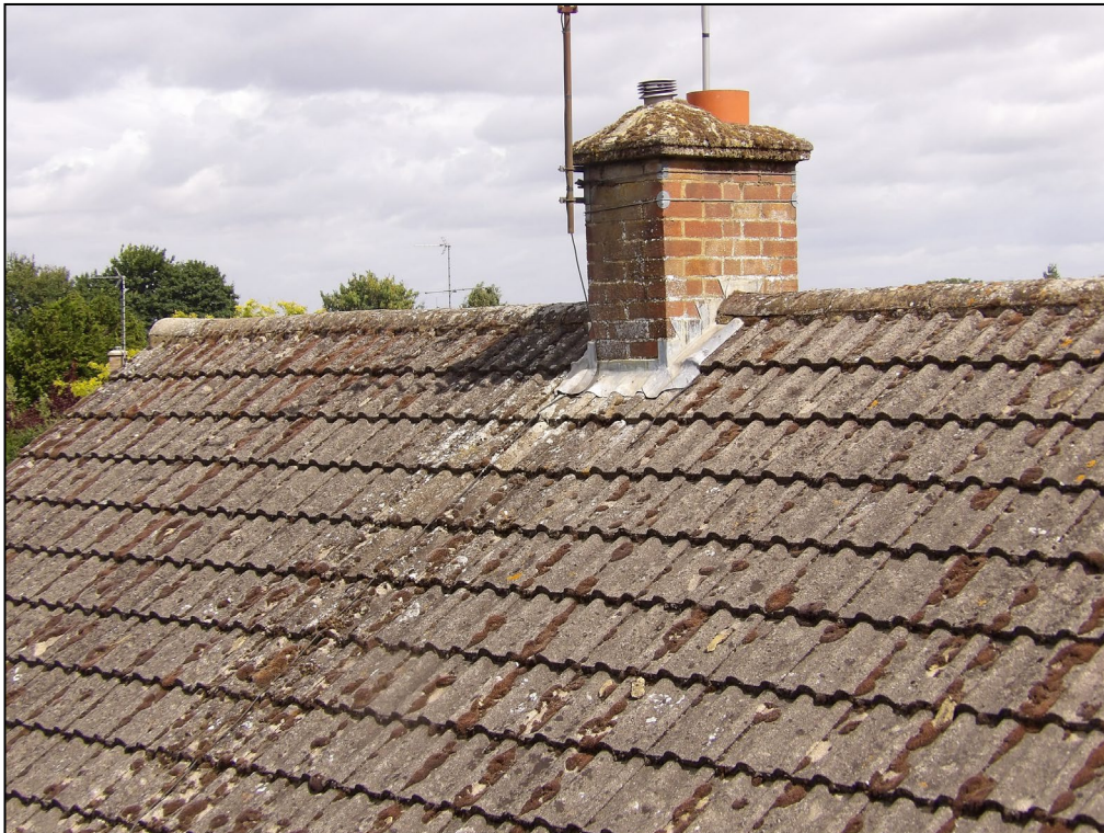
Figure 6. Example of flush lead flashing. 91 London Road, Twyford. 15.07.25
