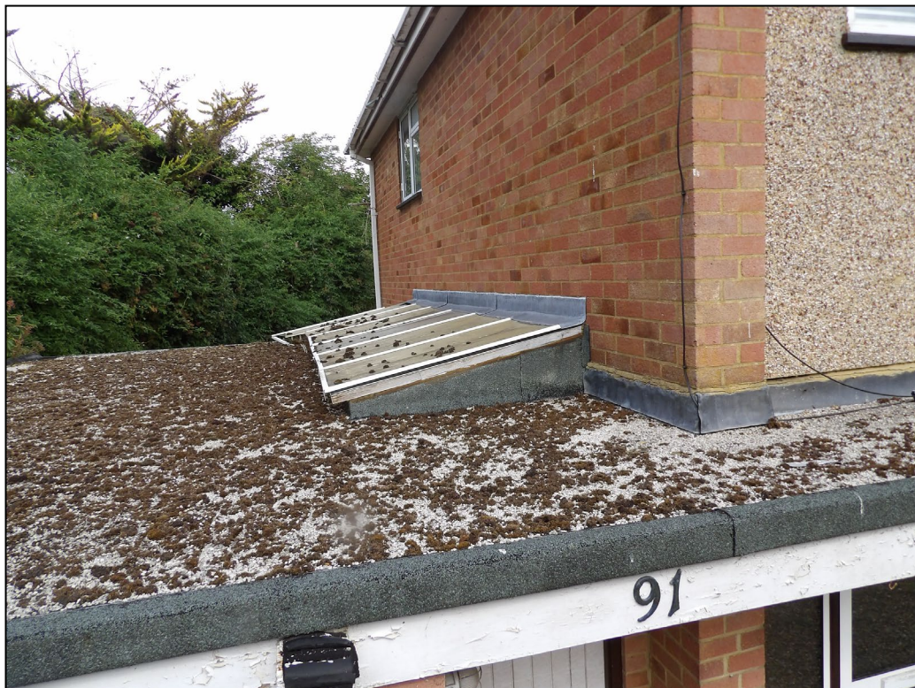
Figure 8. Lightwell and bitumen covered garage roof. 91 London Road, Twyford. 15.07.25
