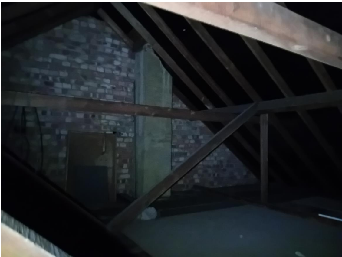
Plate 5: View of the interior loft space
