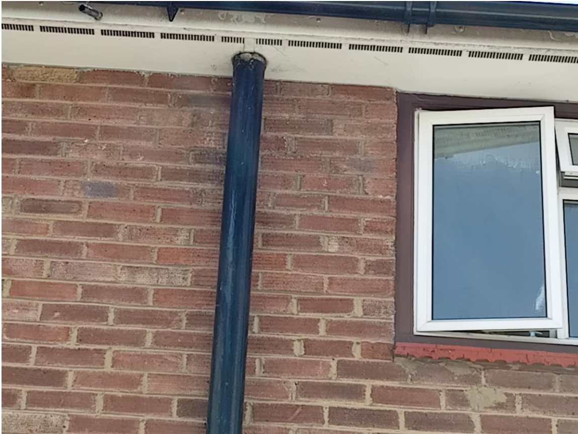
Plate 1: View of the soffit which was found to be in good condition
