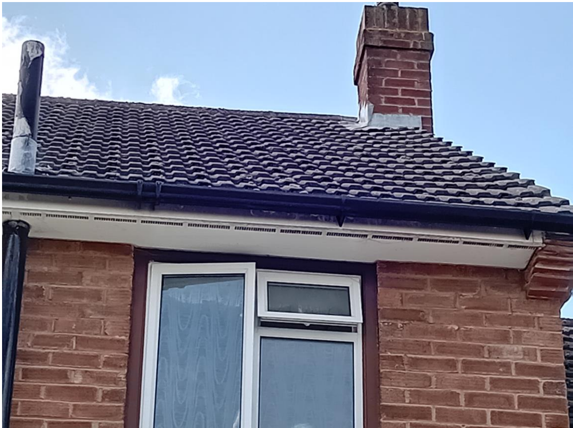
Plate 3: View of the roof tiles at the rear of the property.
