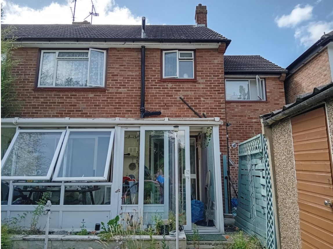
Plate 2: View of the rear elevation
