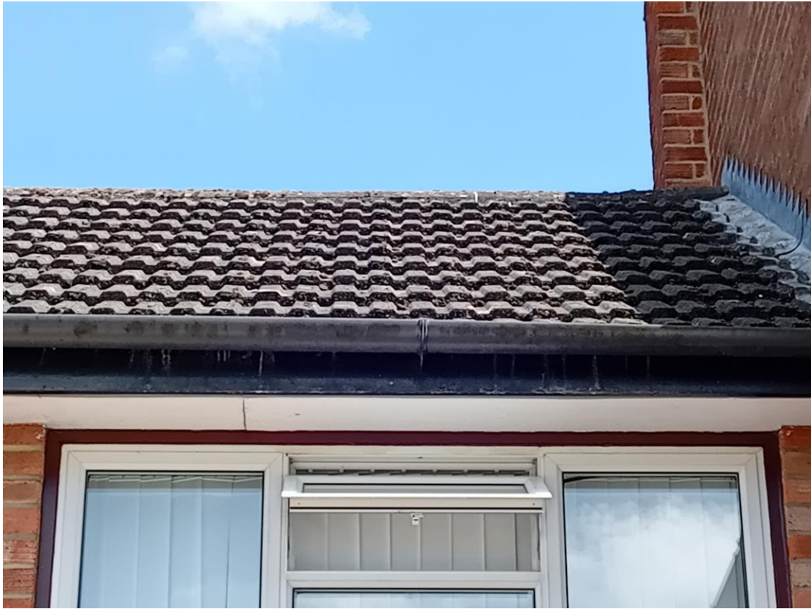
Plate 8: View of the roof tiles at the front of the property.
