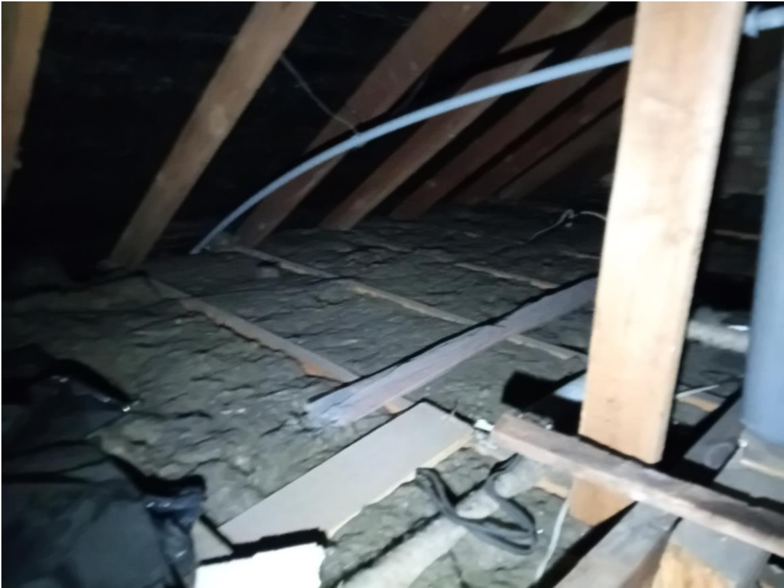
Plate 6: View of the roofing felt and timber beams.
