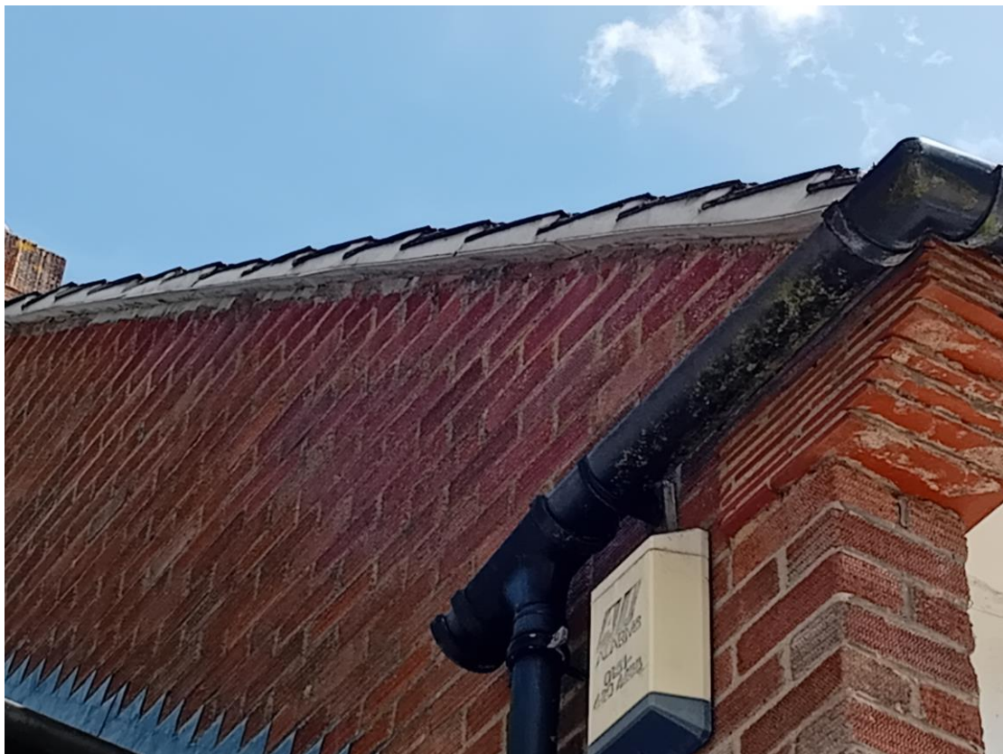
Plate 9: No gaps or missing mortar are apparent on the side elevation.
