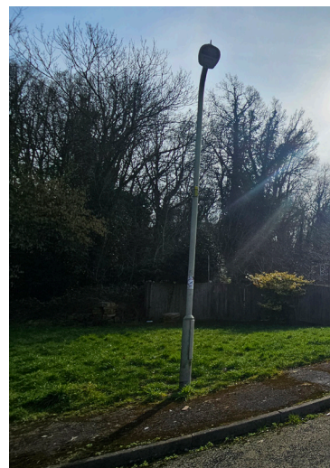
① Existing street lamp
