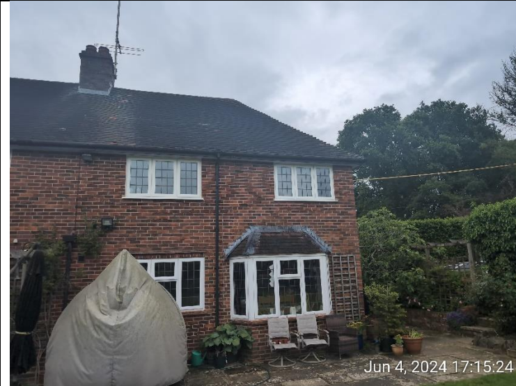
Figure 4: B1 southern elevation with porch. Raised lead flashing circled in red
