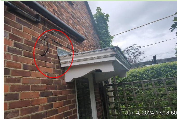
Figure 4: B1 southern elevation with porch. Raised lead flashing circled in red
