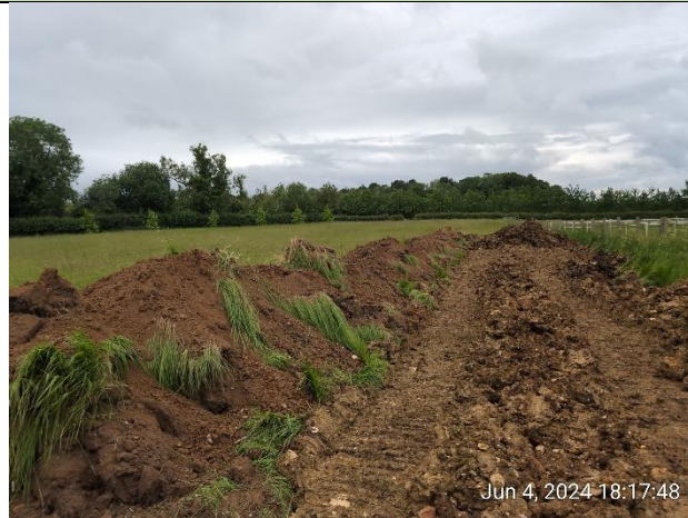
Figure 25: dug earth in western field
