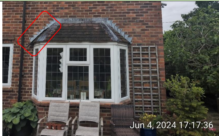
Figure 3: B1 western elevation, bay windows with raised lead flashing
