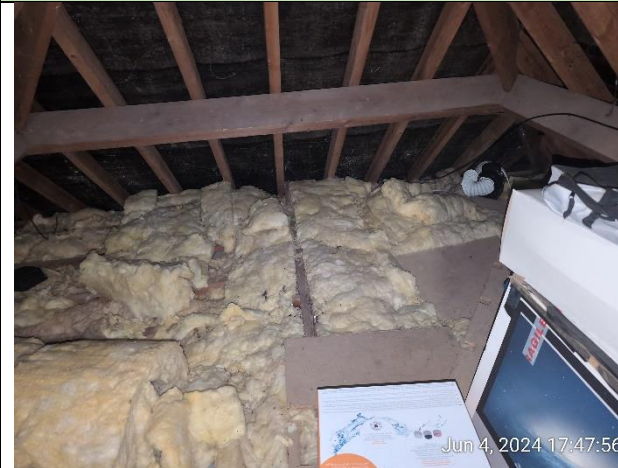
Figure 10: B1 – southern loft space
