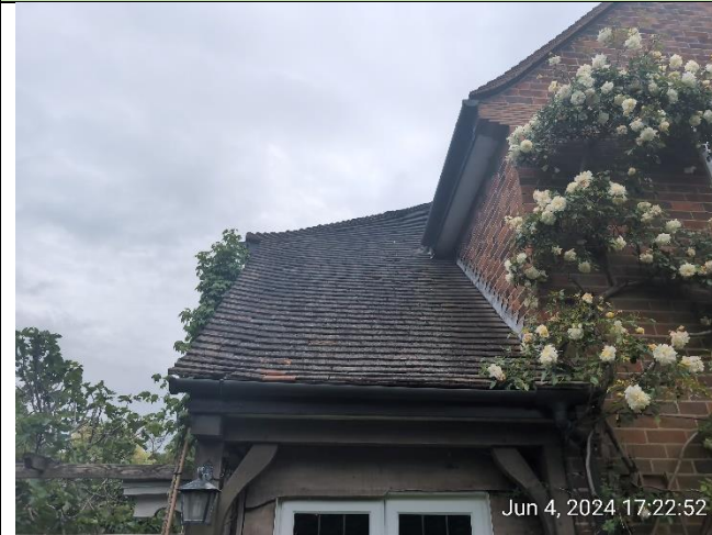
Figure 6: B1 eastern elevation, southern corner
