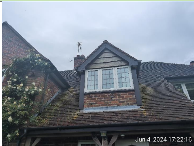
Figure 7: B1 eastern elevation, dormer window
