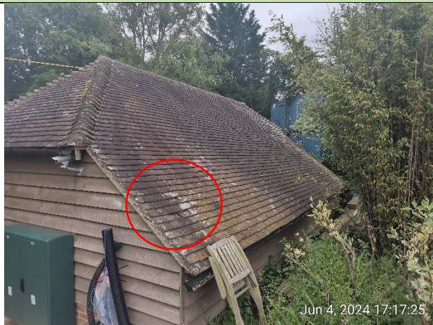
Figure 11: B2 – western elevation
