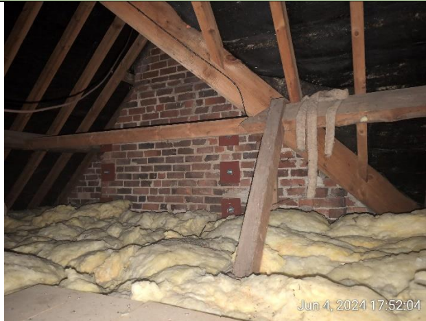
Figure 9: B1 – B1 – northern loft space
