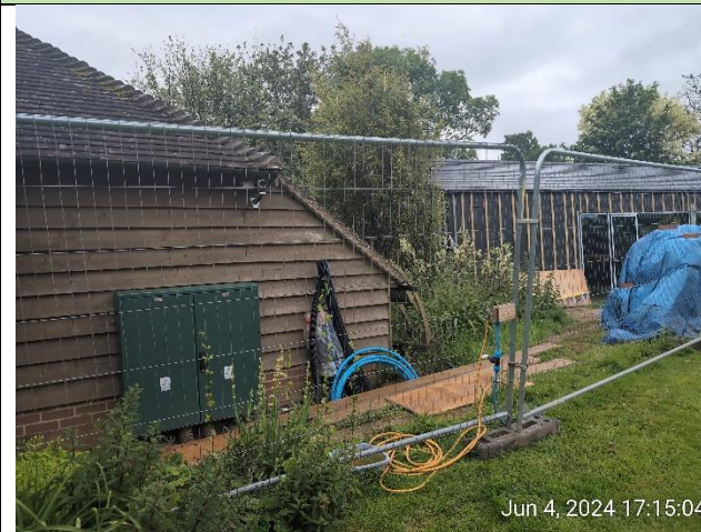
Figure 12: B2 – northern elevation
