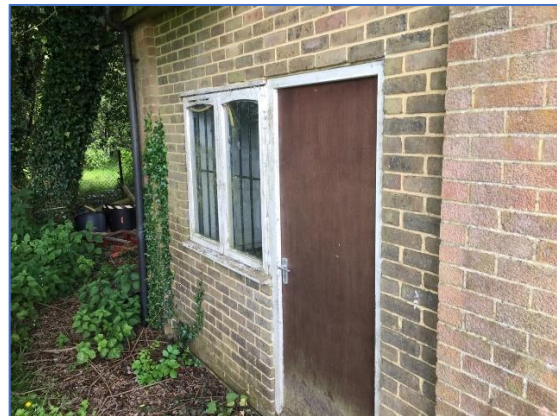
Photo 49 Barn structure (B3)
