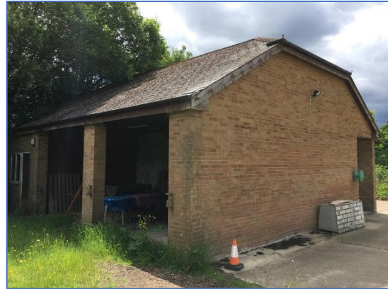
Photo 47 Barn structure (B3)
