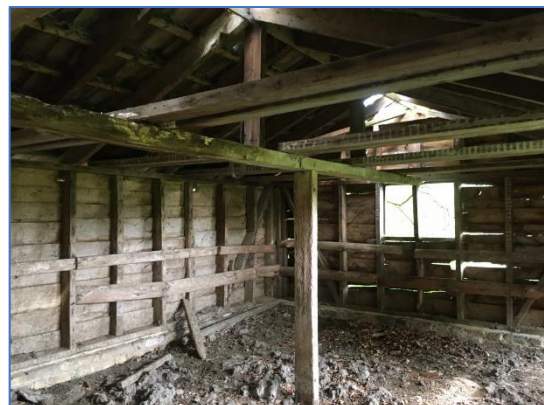
Photo 65 Timber outbuilding internals (B7)
