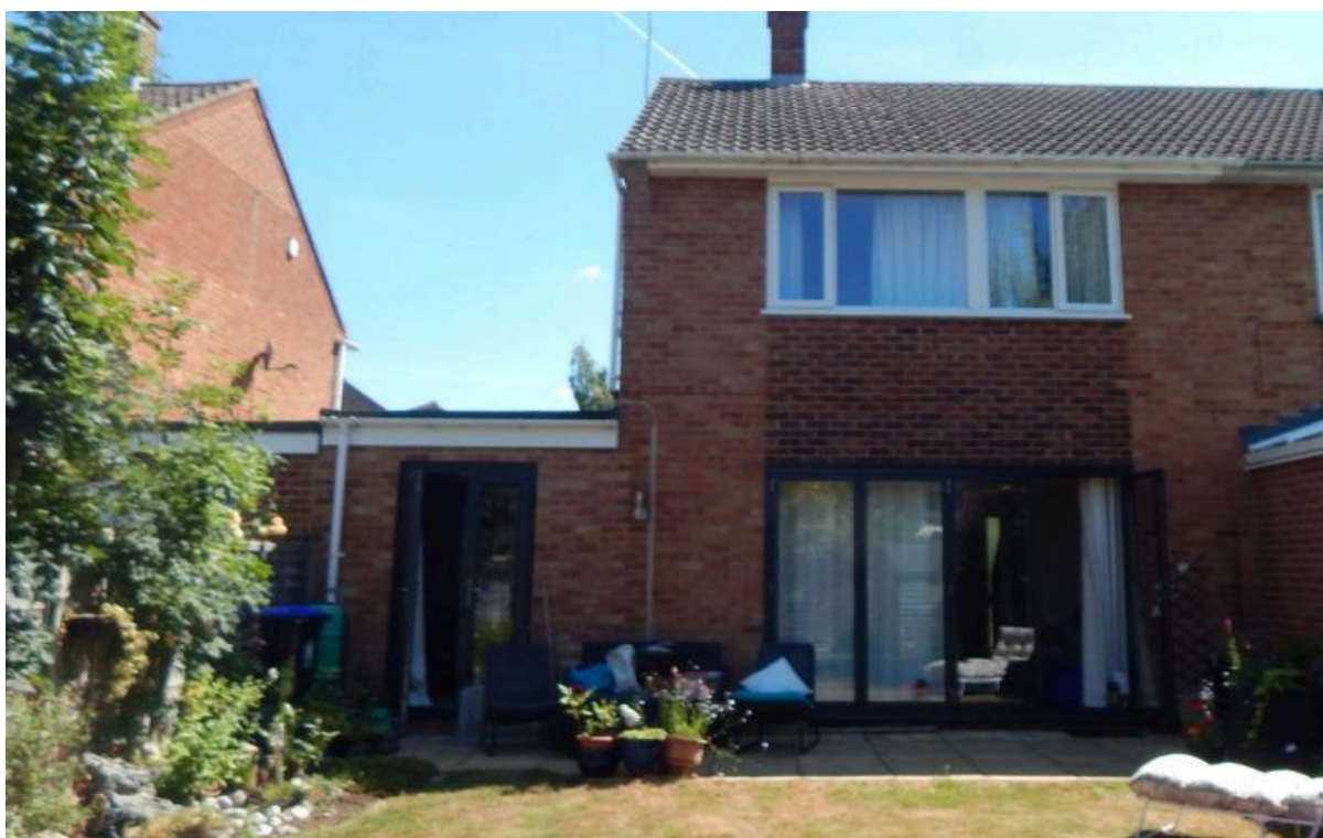
Image 2 – West facing elevation of the property
