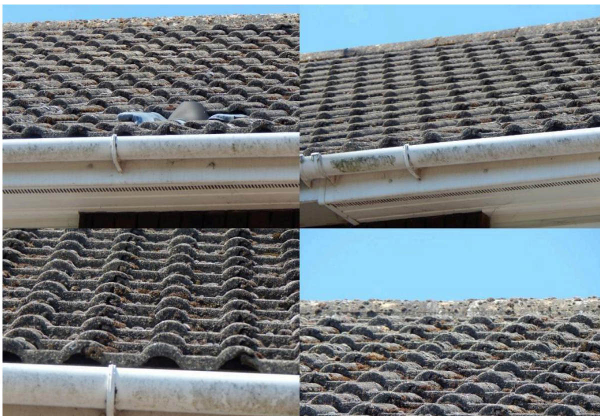
Image 5 – Close view of main tiled roof coverings to demonstrate example of condition
