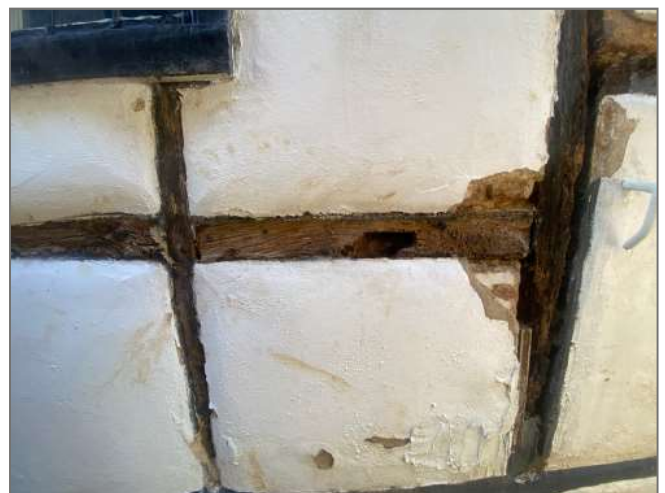
Fig. 3: Close up of S3 stud and two rails
