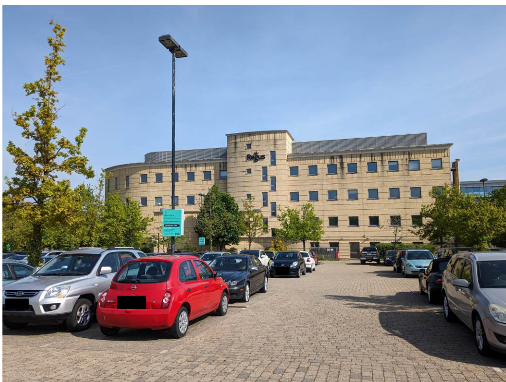
Photograph 6 – View from building from south-east corner of site
