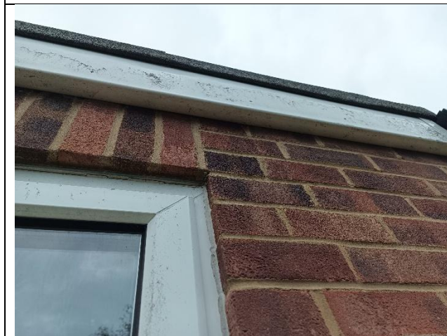
PHOTOGRAPH 11- WELL SEALED FASCIA
