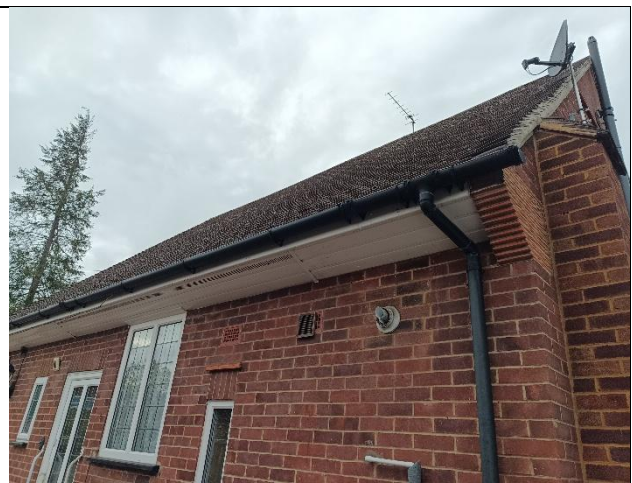
PHOTOGRAPH 6– WELL SEALED SOFFITS AT THE EAVES
