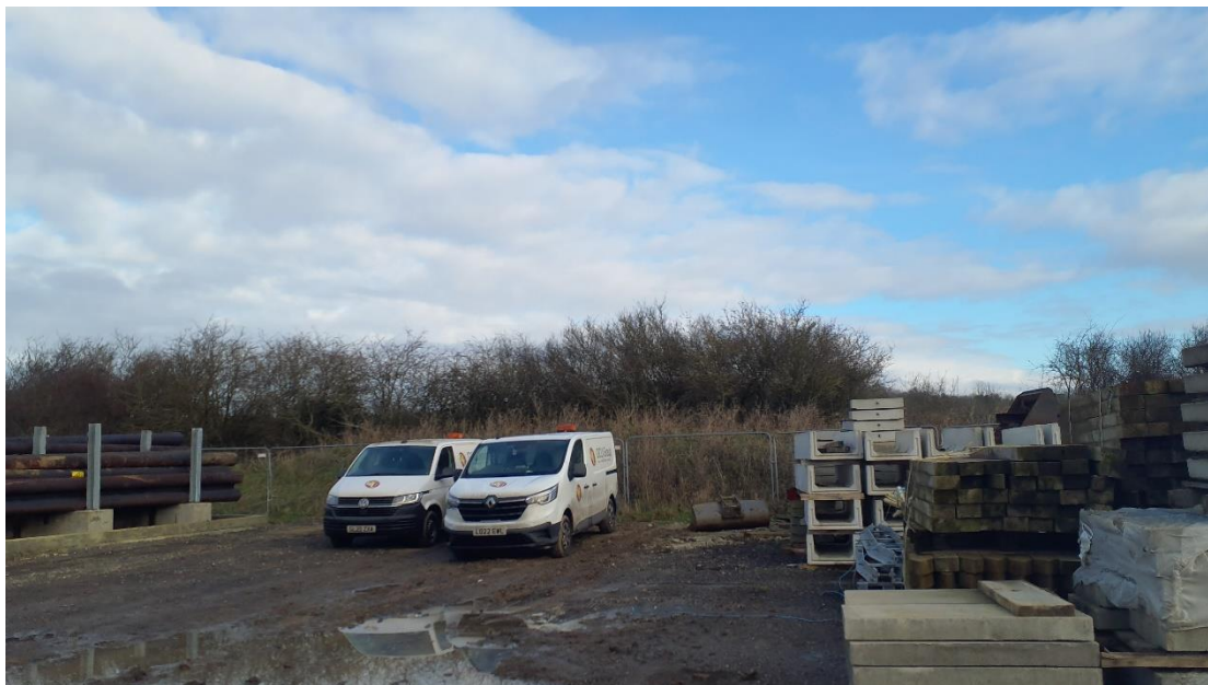
Figure 9 – The north-eastern corner of the site, pictured from the south-west. No trees pictured are close enough to the compound to be affected by its retention.
