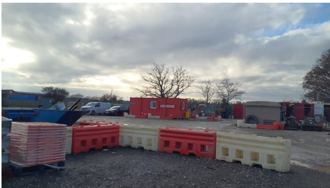
Figure 12 – The western boundary of the site, pictured from the north-east. T14 is visible centre frame, with T13 and T12 to its right, and T11 just visible on the far right.
