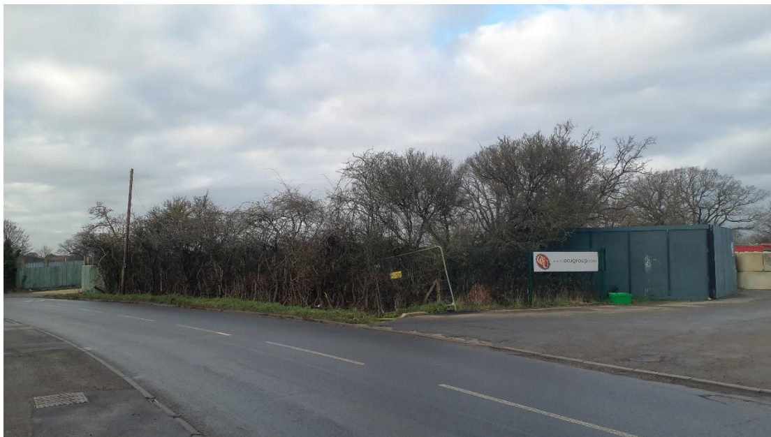
Figure 3 – The southern boundary of the site, from the entrance to the south-western corner. T5 is visible by the entrance, with G2 running along the verge and T6 visible to the left of the telephone pole.
