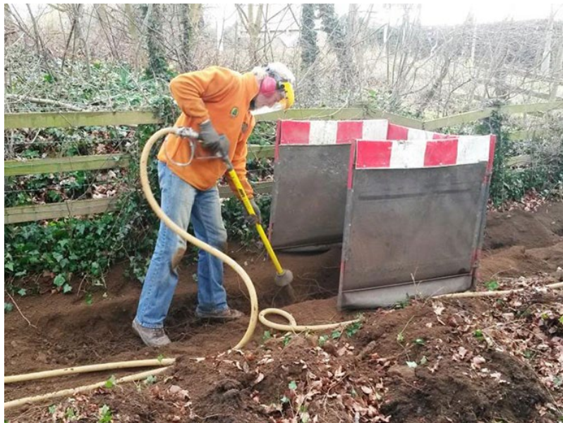
Image of an Air Spade in operation.
