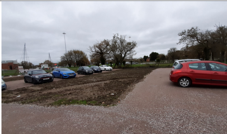
Figure 1 Hardstanding and parked cars substantially complete. Image taken 17th November 2020
