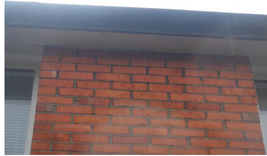
Photograph 7. Tight timber soffits and fascia's (southern elevation).
