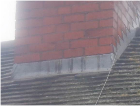
Photograph 6. Lead flashing around chimney flush to plain roof tiles (northern elevation).
