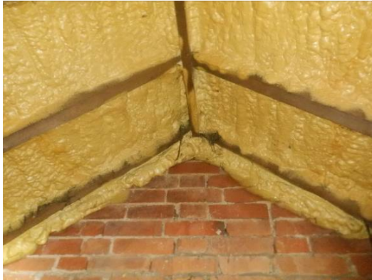
Photograph 10. Roof void with roof covered by spray foam insulation.
