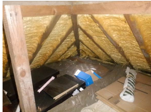
Photograph 12. Spray foam insulation filling eaves (roof void).
