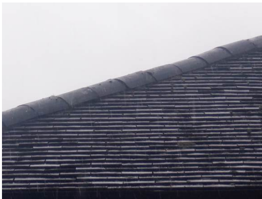
Photograph 3. Flat plain roof tiles and fully mortared hip (northern elevation).
