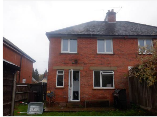
Photograph 2. Rear of property viewed from north.
