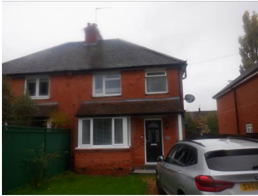
Photograph 1. Front of property viewed from south.
