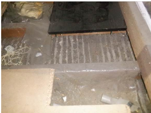
Photograph 13. Plastic sheeting on floor of roof void covering the joists (roof void).
