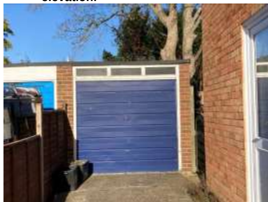
10. The garage viewed from the front (south east).
