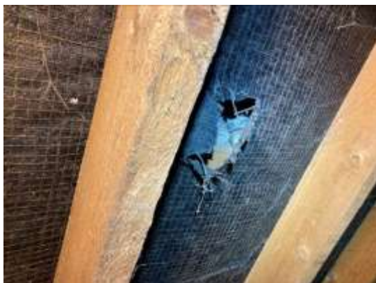
15. One of the tears in the felt.
