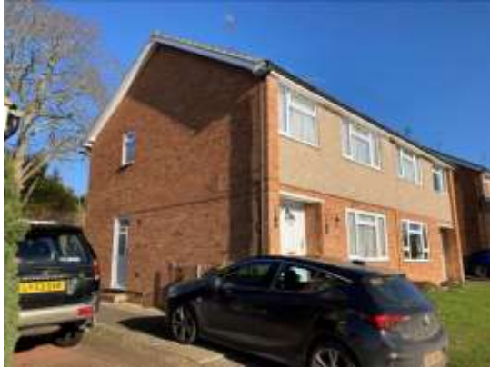
1. The house viewed from the front (south east).
