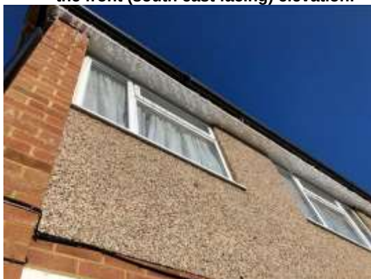
9. Tightly fitted uPVC soffits to the front.
