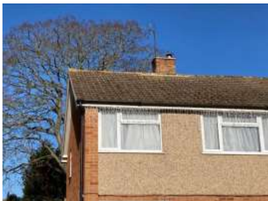
7. The mostly tightly fitted concrete tiles of the front (south east facing) elevation.
