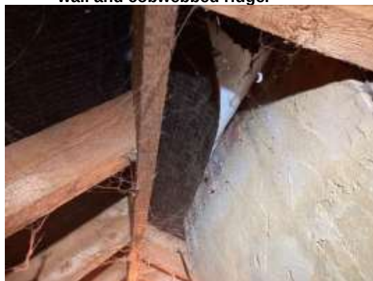
16. A section of breathable roofing membrane (BRM) filling a gap around the chimney.
