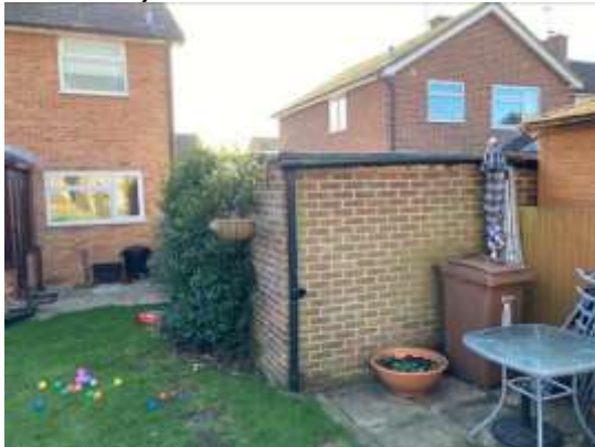
3. The garage viewed from the rear.
