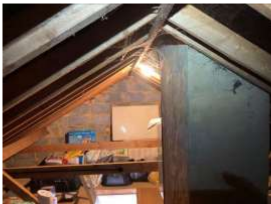
13. The house loft showing cement covered chimney.
