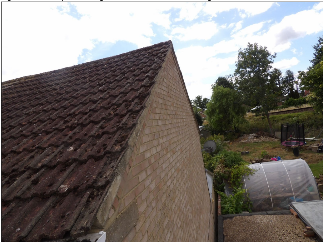
Figure 6. Example of verges. 5 Brook Close, Wokingham. 30.07.25
