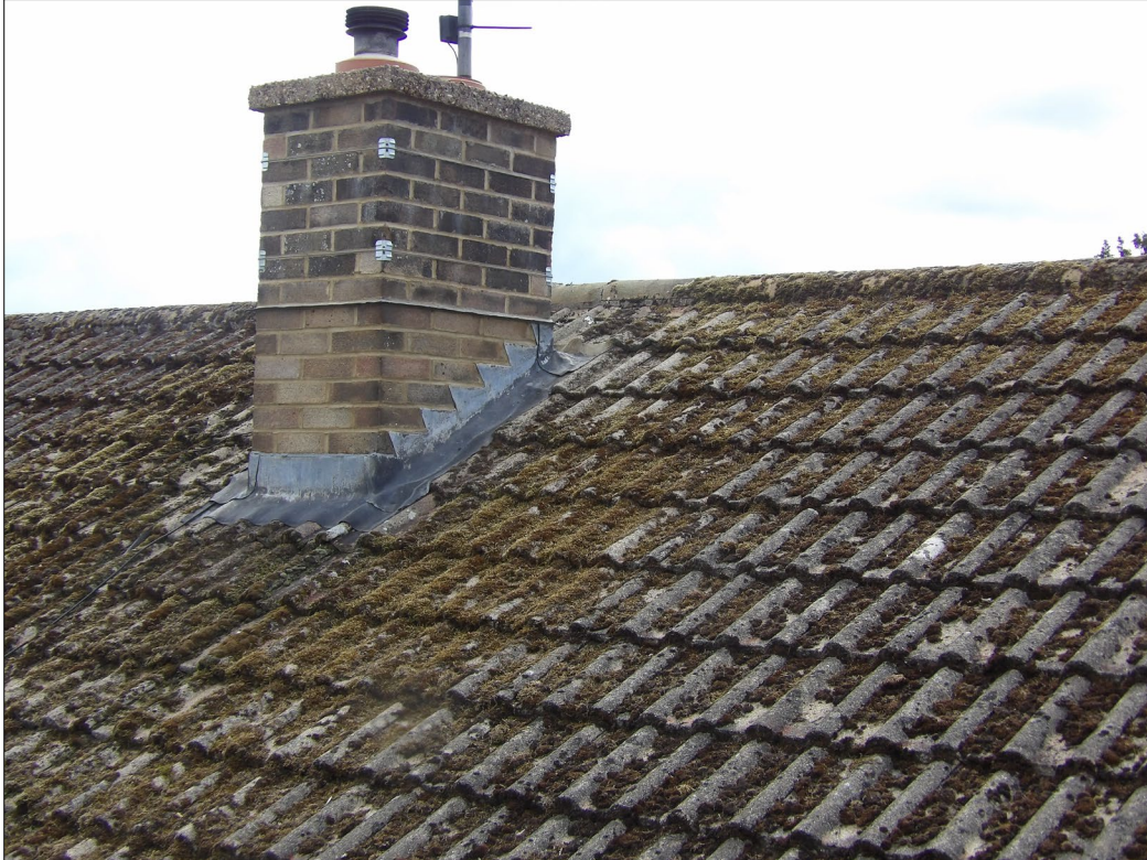
Figure 5. Example of ridge tiles and lead flashing. 5 Brook Close, Wokingham. 30.07.25
