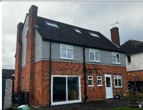
Figure 2: East and southern elevations of B1
