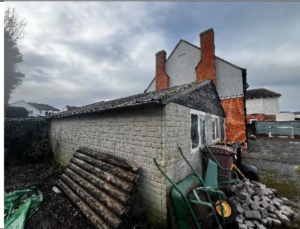
Figure 11: South and east elevations of B2
