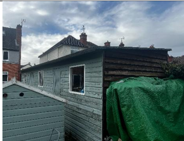
Figure 14: East and south elevations of B3
