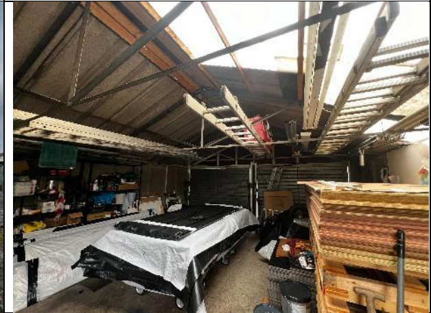
Figure 12: Interior of B2
