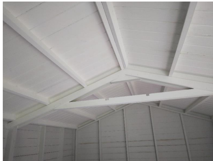
Building B3 (no evidence – negligible roost suitability)
