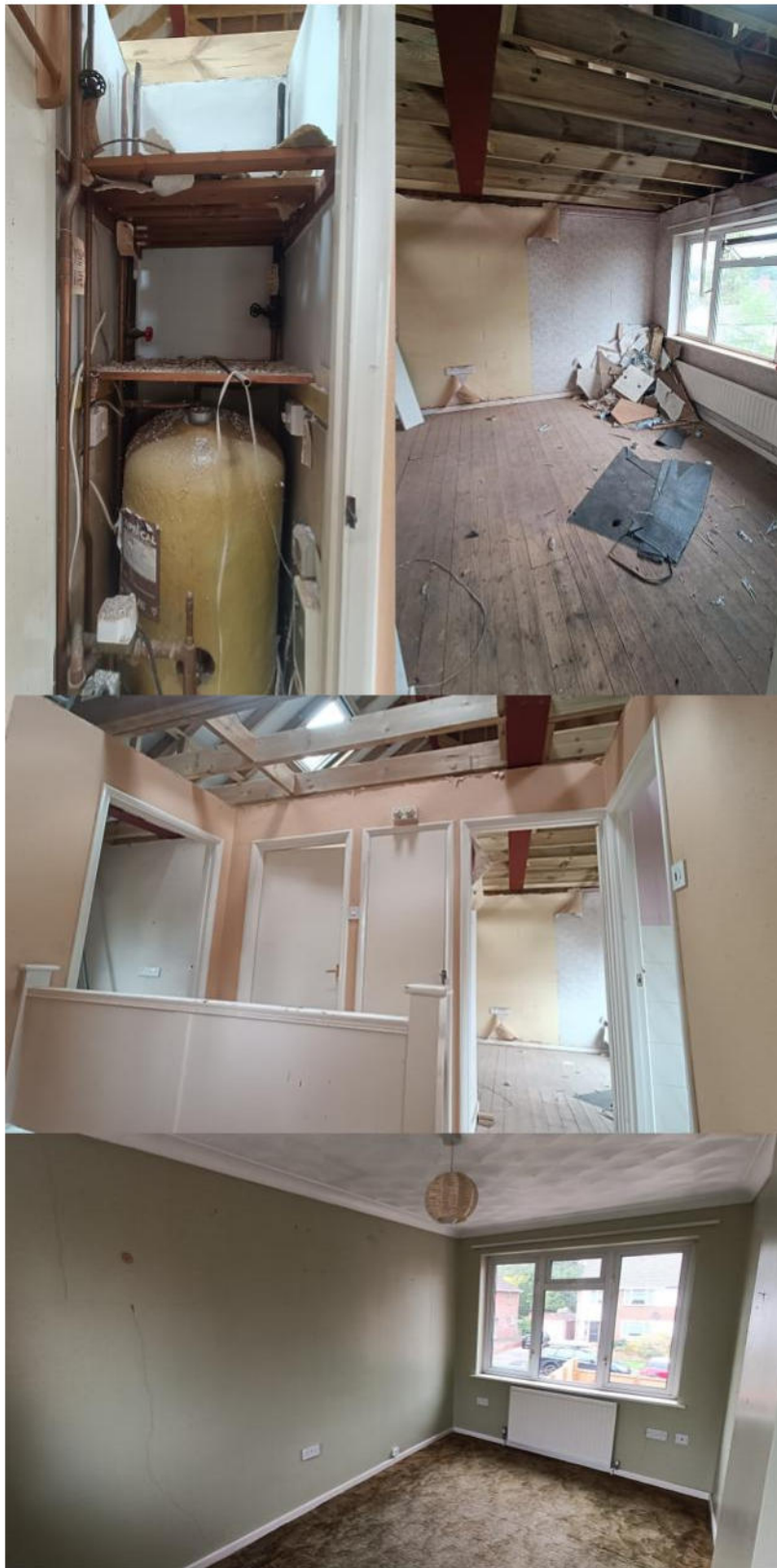
Upper Left: 1 st floor landing boiler / airing cupboard. Upper Right: 1 st floor bedroom interior. Middle: 1 st floor landing. Bottom: 1 st floor extension interior.
