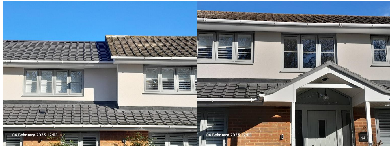
Good condition, flat fitting roof tiles, well sealed windows, and mortar at verges intact (both).
