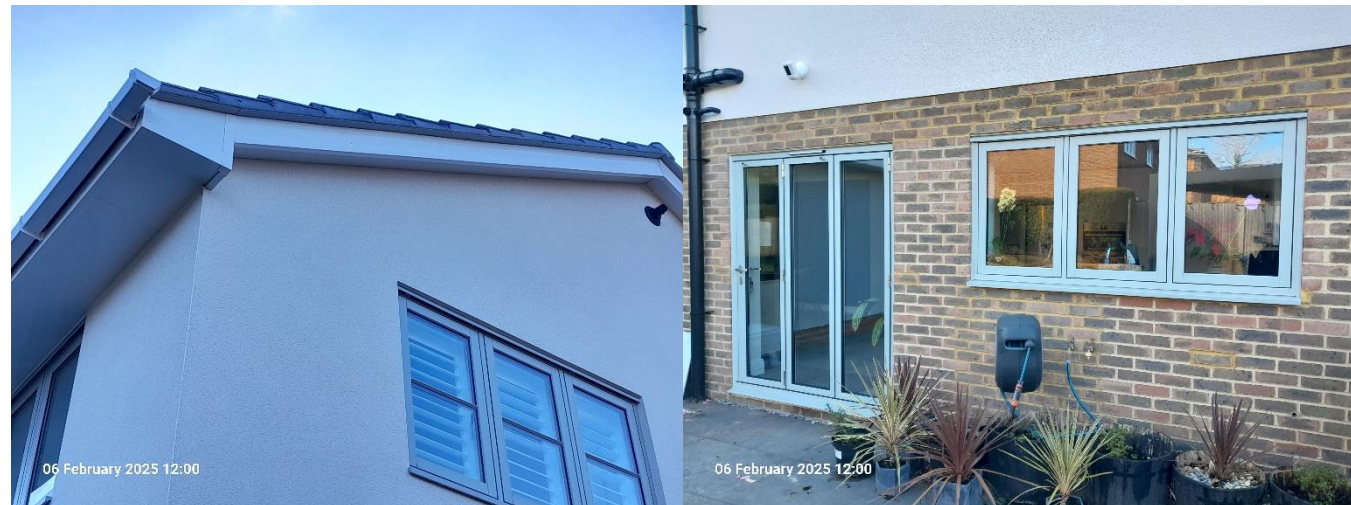
Well sealed soffit, render, and mortar (left) and tight fitting doors and windows with brickwork and mortar intact (right).
