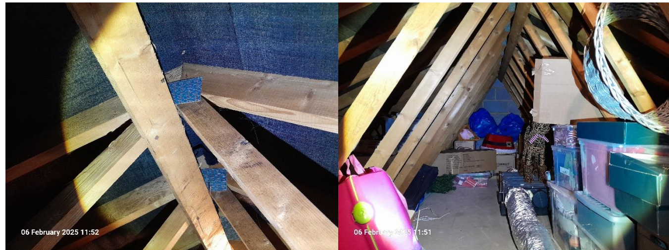
Bitumen felt in good condition, no central ridge beam (left) and the loft void (right).
