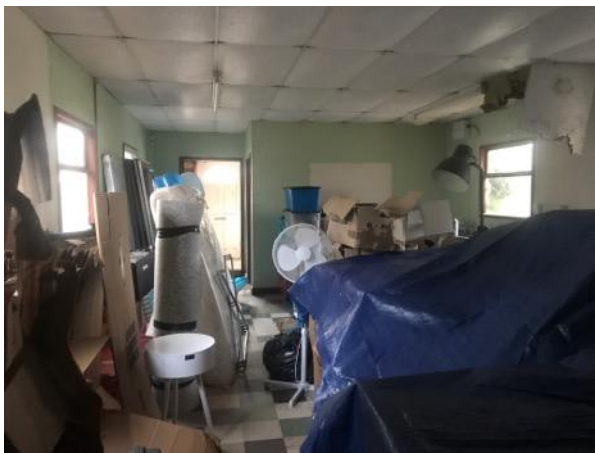
Photo 9: Interior of building B1
