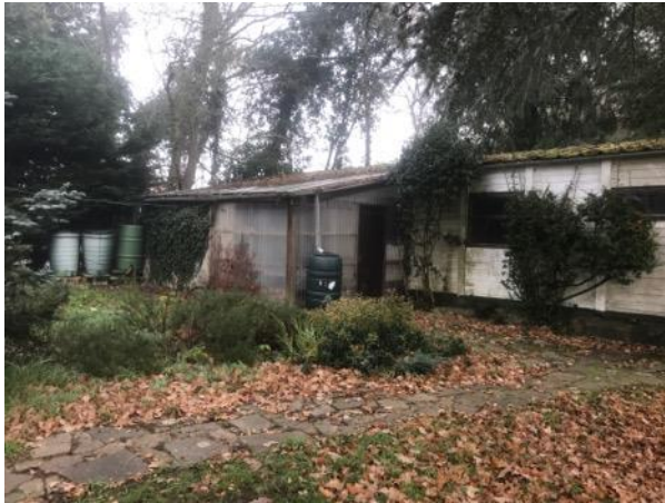
Photo 7: West elevation of building B1
