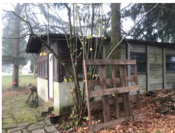
Photo 6: East elevation of building B1
