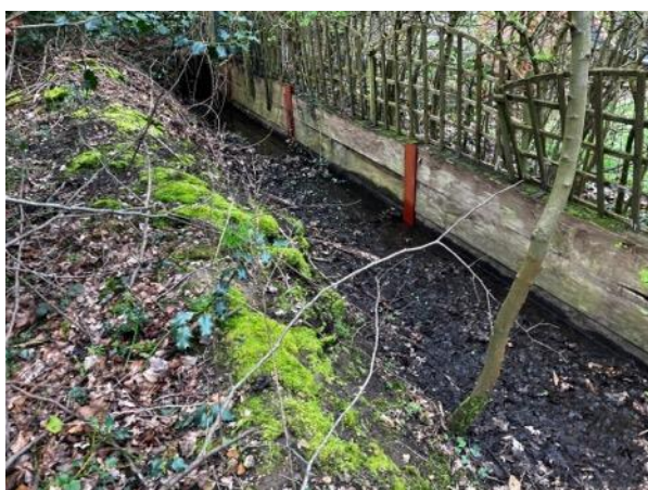
Photo 5: Ditch in north of the site
