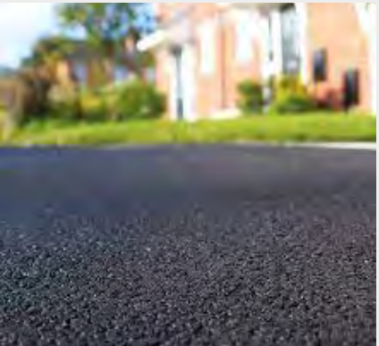
Macadam surfacing with flat top concrete edging
