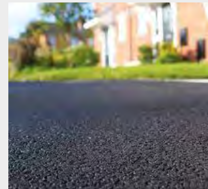
Macadame surfacing with flat top concrete edging
