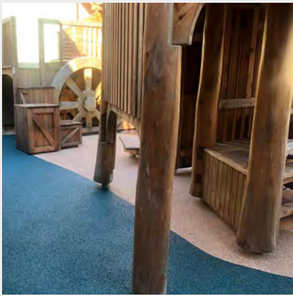
Wet pour safety surfacing Colour: Mixture of buff, red and blue Example shown: RubbaSmart by Play Smart UK
