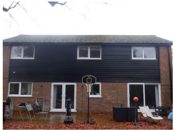
Photograph 2. Rear elevation of the house, viewed from the north.
