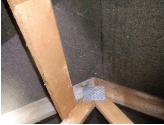
Photograph 8. Cobwebbed rafters with no ridge beam (roof void).
