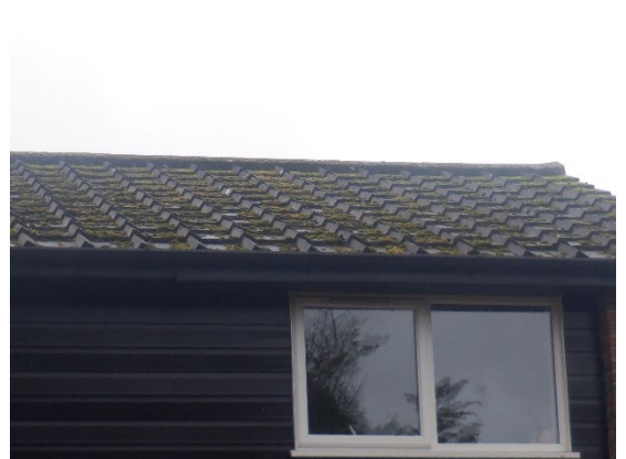
Photograph 4. Intact ridge tiles (rear elevation).
