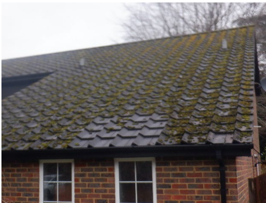
Photograph 3. Tight, mossy interlocking roof tiles (front elevation).
