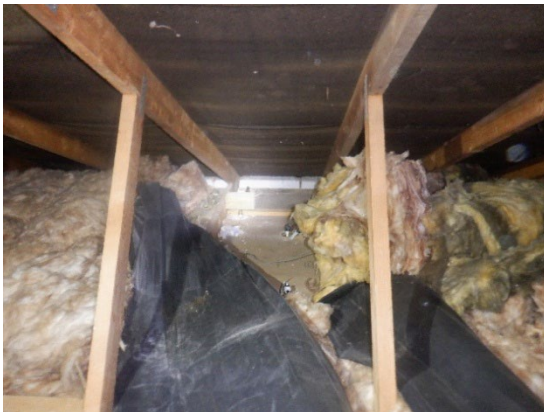
Photograph 10. Fibreglass insulation up to open eaves (roof void).
