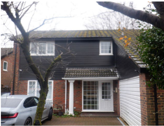
Photograph 1. Front elevation of the house, viewed from the south.
