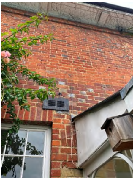
Figure 12: Blocked window openings on the left hand side of the rear elevation
