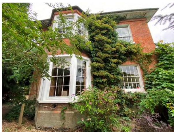
Figure 9: 2-storey canted bay on the north-east elevation
