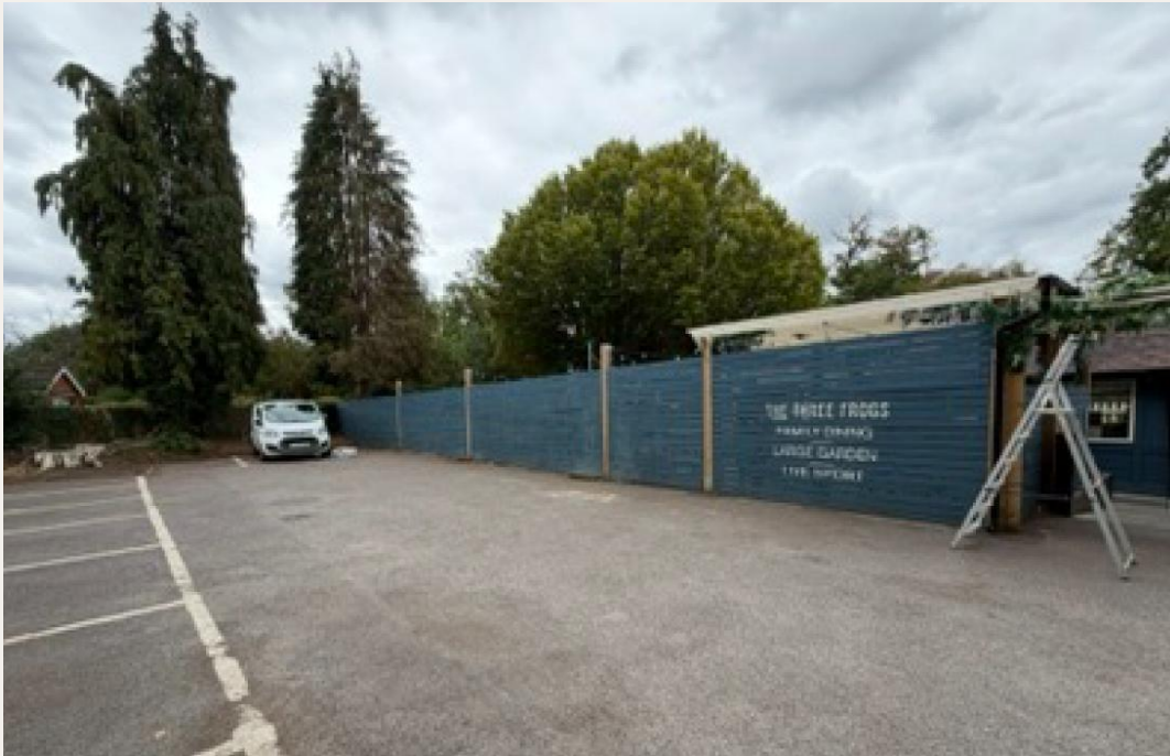
Figure 4 Extended fence around pub garden - now having been fully painted blue as of 10 th September 2026
