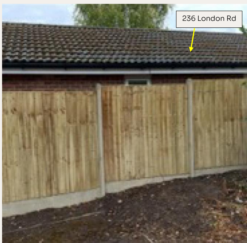
Figure 8 Photos of new extended height fencing bordering the neighbour
