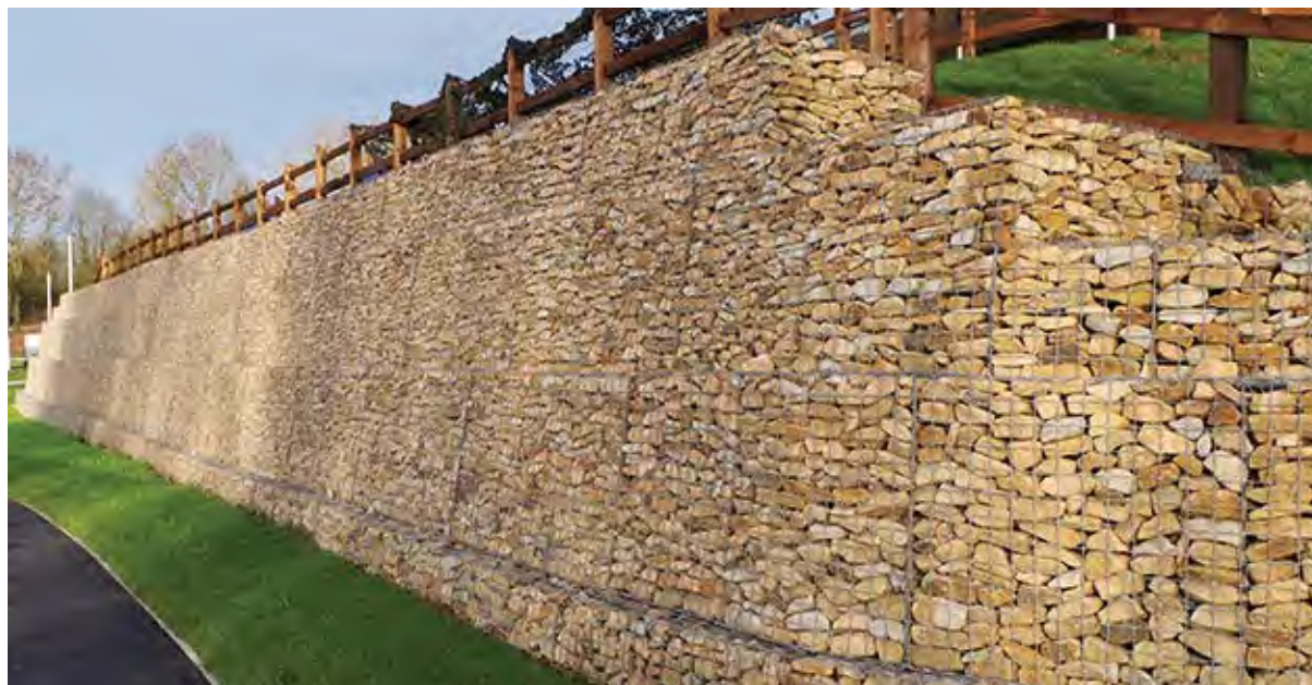
Enviromesh designed, supplied and installed the above stepped-face gabion retaining wall at the Beacon Barracks MoD site in Stafford. For more information on this Case Study, please visit our website: enviro-mesh.com
