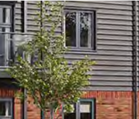
Timber cladding
