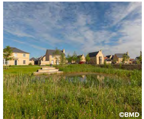
Houses overlooking SuDS pond
