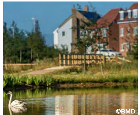
Houses overlooking SuDS pond
