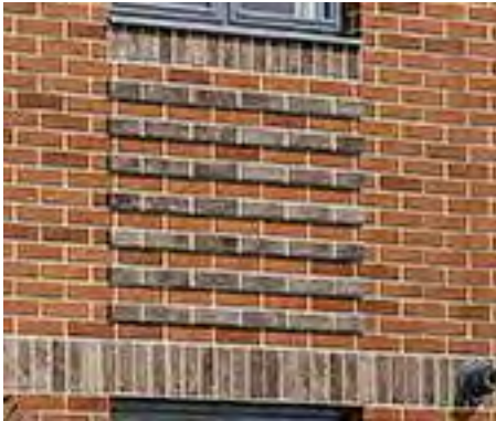
Projected brick work feature
