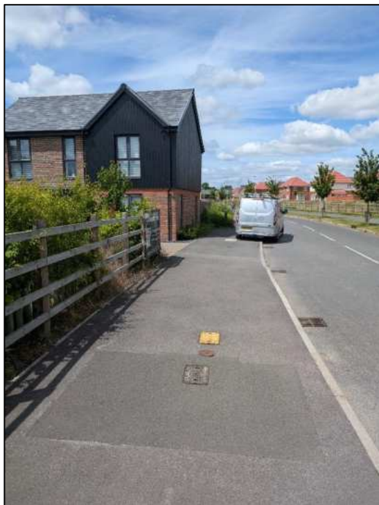
Image 6.1 Footway/cycleway provision along Princess Marina Drive
