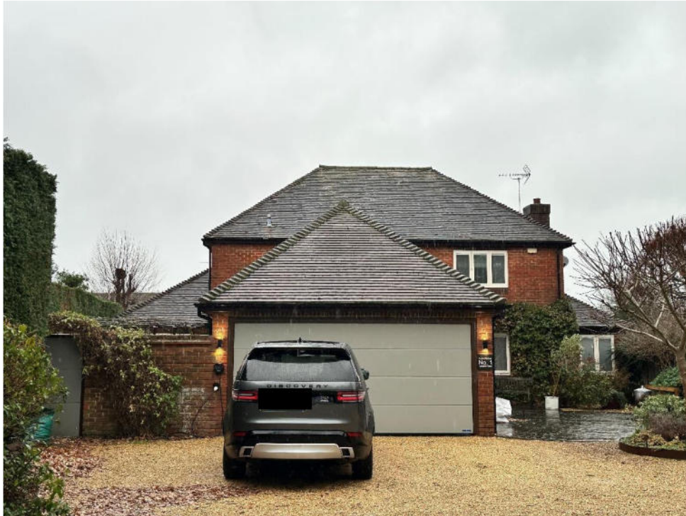
STREET VIEW OF 1 ORCHARD PLACE
