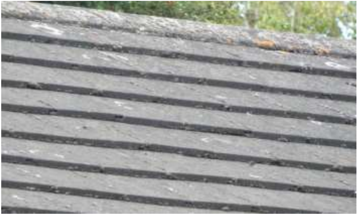
Image 5 – Close view of the main roof coverings to the dwelling
