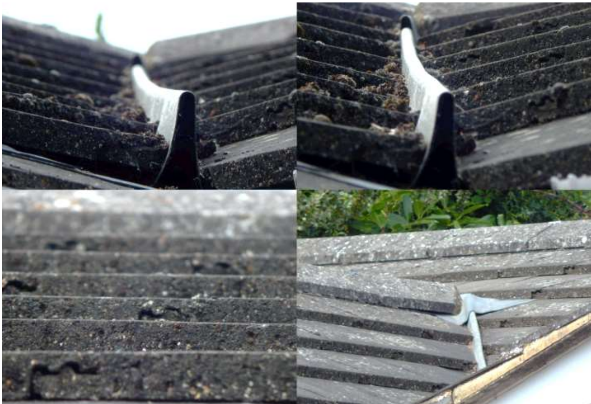
Image 6 – Close view of the main roof coverings to the dwelling
