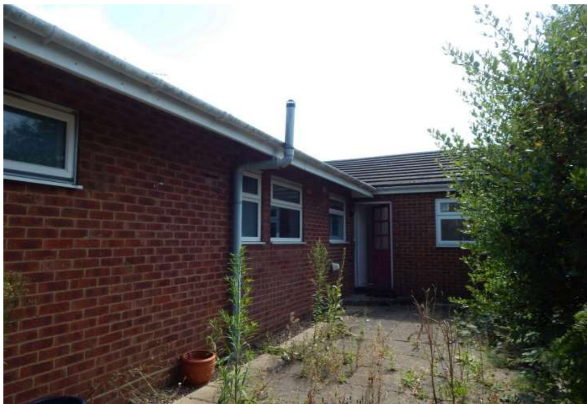
Image 3 – West facing elevation of the dwelling
