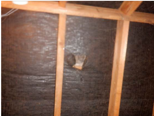
15. One of the tears in the felt.
