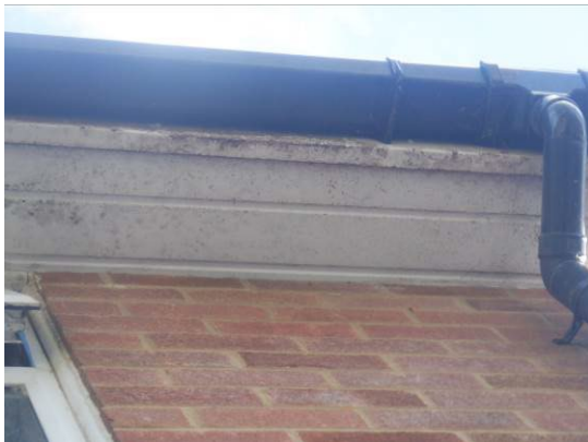
5. The tightly fitted uPVC soffits to the rear.
