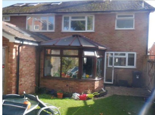
2. The house viewed from the rear (north west).
