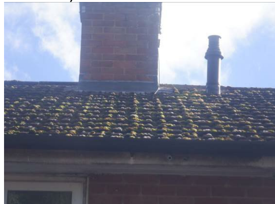
4. The tightly fitted concrete roof tiles and lead flashing around the chimney.
