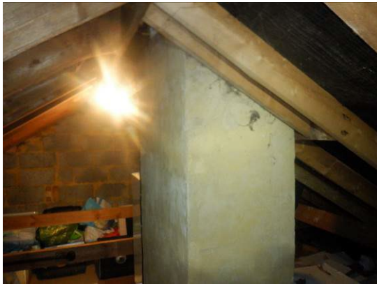
13. The house loft showing cement covered chimney.
