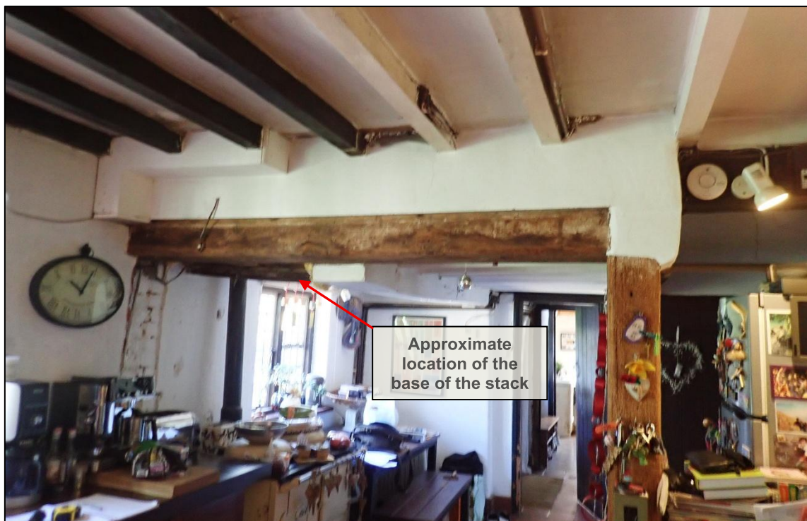
Figure 5. View of the chimney stack at the rear of the property.
