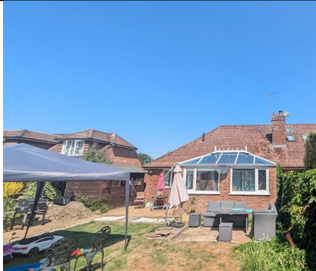
South-easterly rear of the building.
