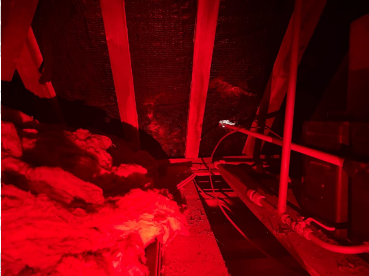
Photograph 11. Internal loft void showing exposed roof timbers, underlay, insulation, pipework and services. The inspection identified no visible evidence of roosting bats within the accessible area; however, concealed voids behind insulation, underlay, roof tiles and inaccessible roof interfaces could not be fully inspected without intrusive works.
