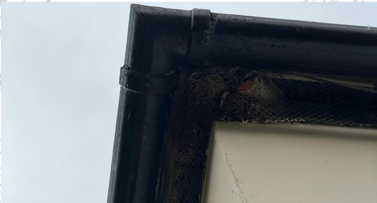
Photograph 6. Eaves and fascia/soffit area showing open and irregular gaps behind the gutter line and beneath the roof edge, suitable for crevice-dwelling bats.
