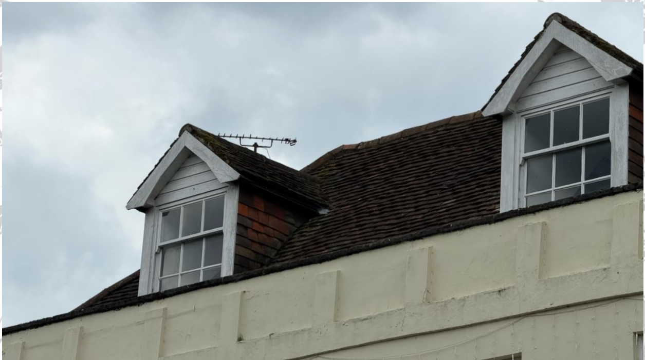
Photograph 8. Wider roof elevation showing multiple dormer structures, clay-tiled roof slopes, ridge and hip features, and widespread potential crevice opportunities.
