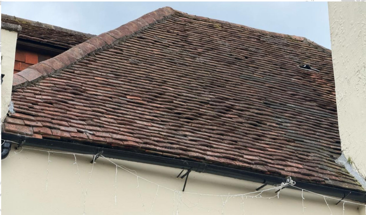
Photograph 2. Roof slope adjacent to chimney structure showing uneven roof tiles, gaps beneath tiles, eaves features and potential access opportunities along the roof edge and gutter line.
