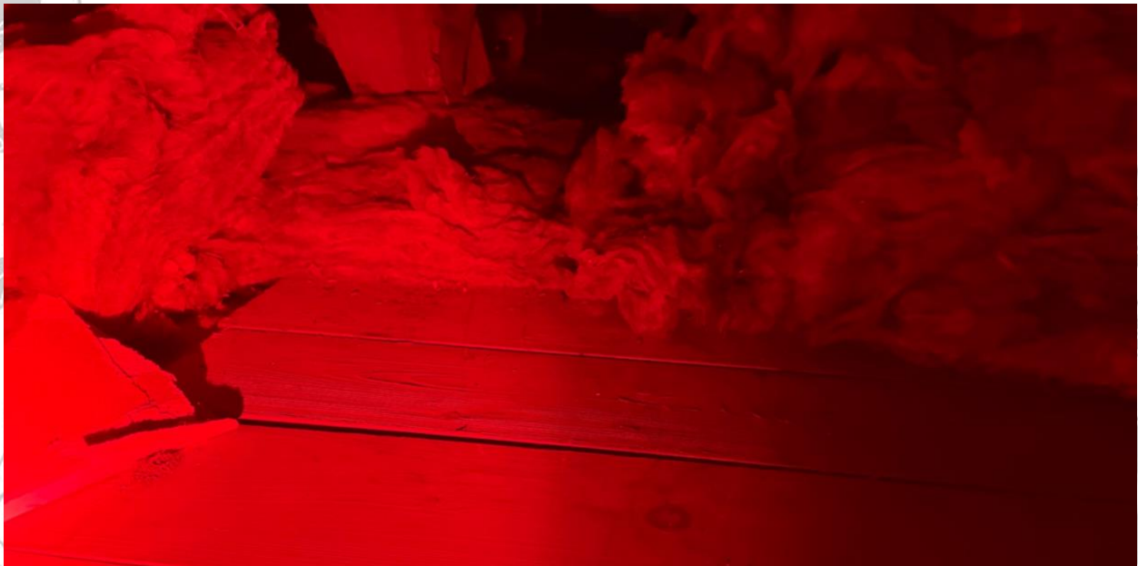
Photograph 10. Internal loft inspection area showing timber boarding, insulation and concealed roof void spaces. No visible evidence of bat use was recorded in the accessible inspection area, including no bat droppings, feeding remains, staining, live bats or dead bats.
