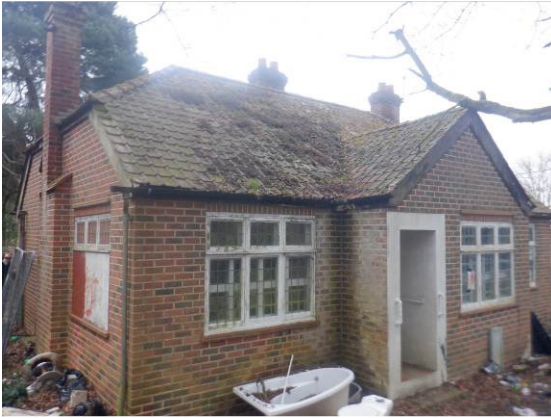
Photograph 1. Front of property viewed from north.
