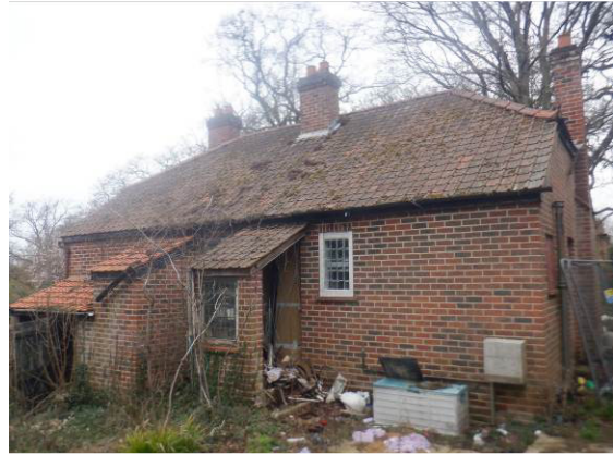
Photograph 2. Rear of property viewed from south.
