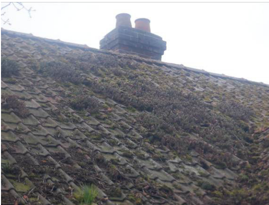
Photograph 3. Interlocking clay tiles (front elevation).
