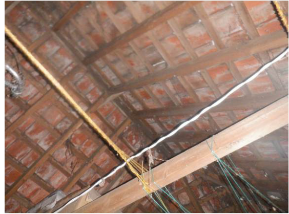
Photograph 12. Unlined roof (roof void).
