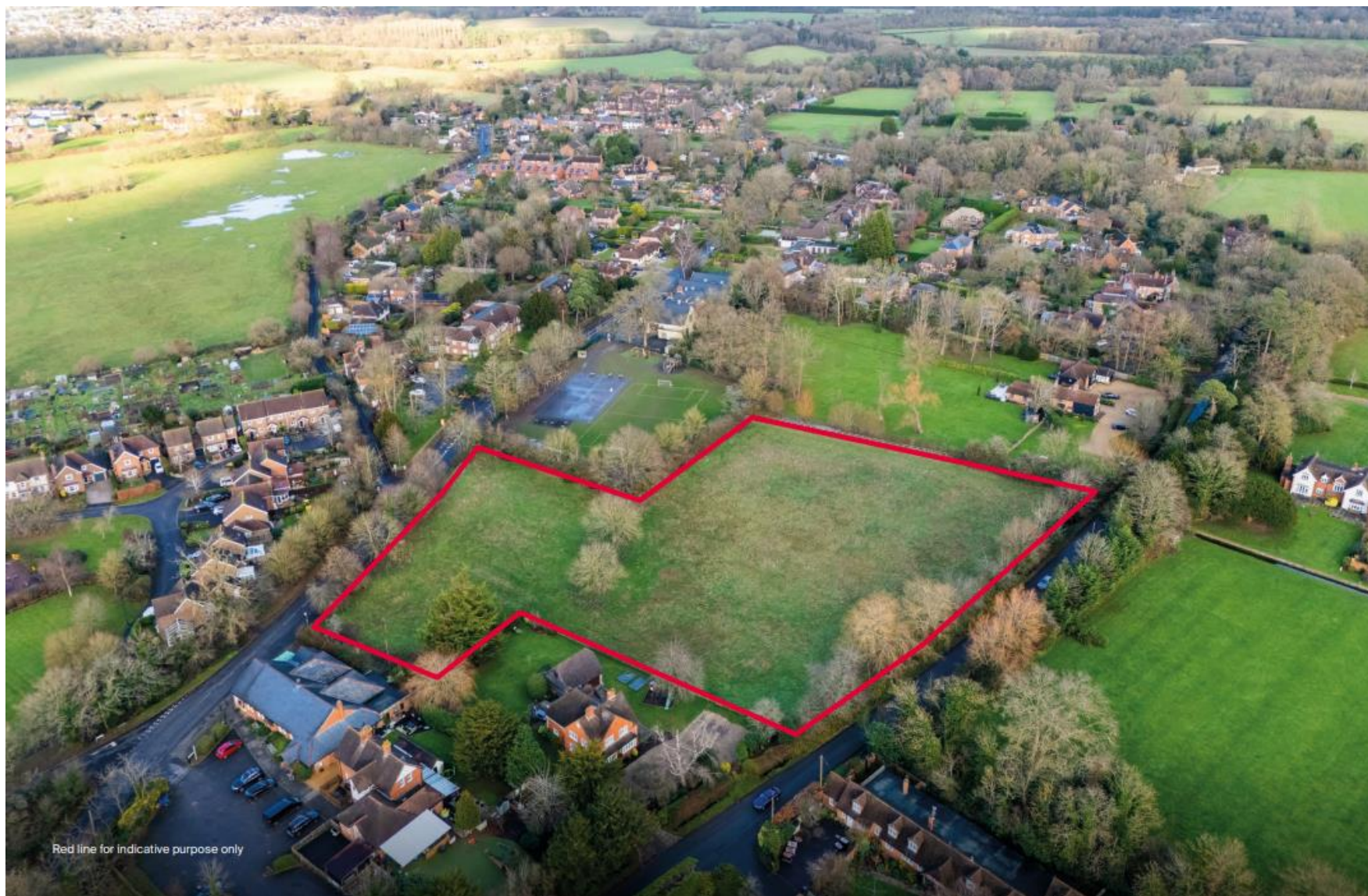
Fig. 1 Aerial view of the development area
