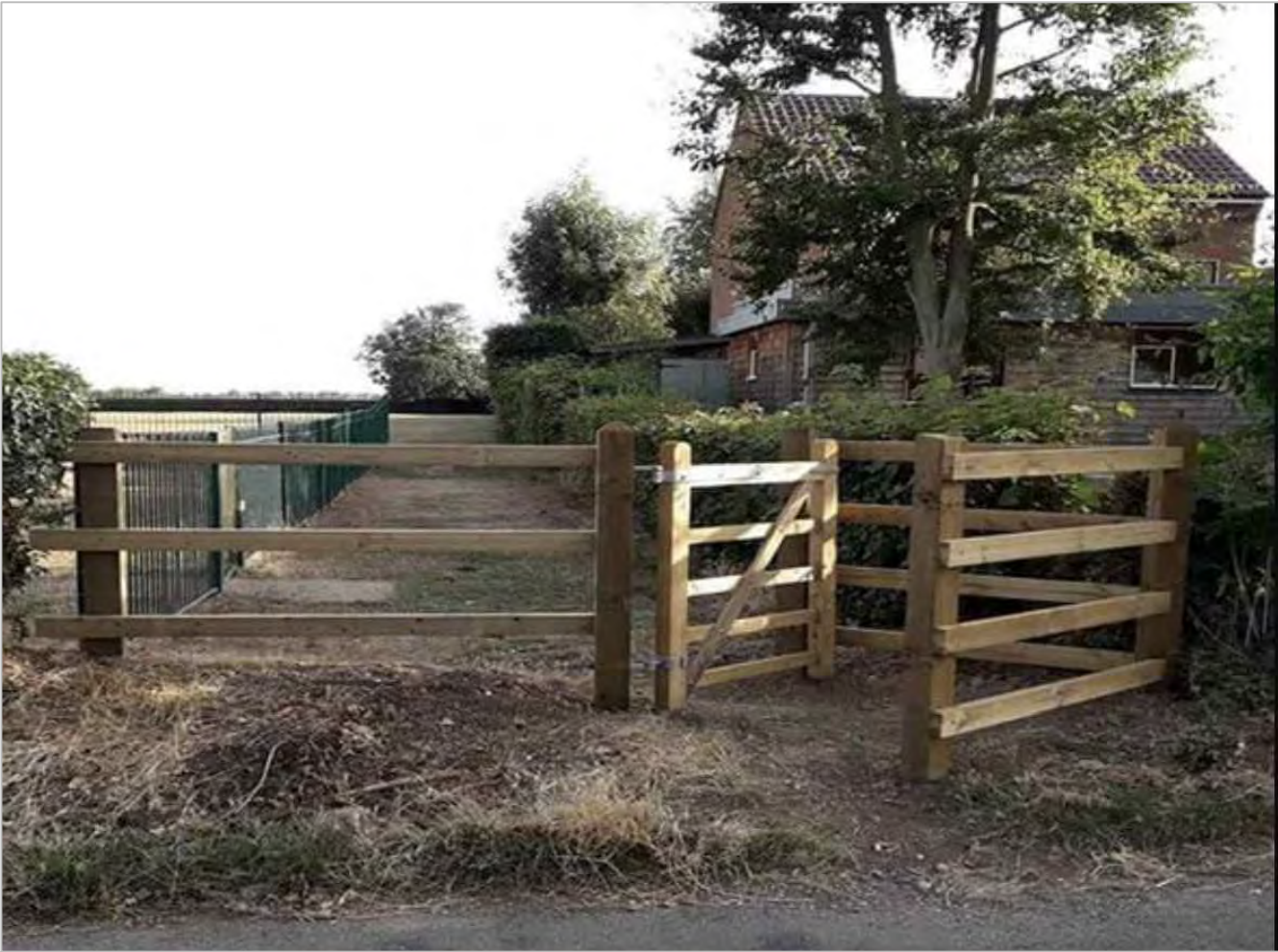
Timber Kissing Gate
