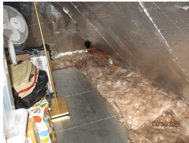
Photo 11: Internal of Void 1.
