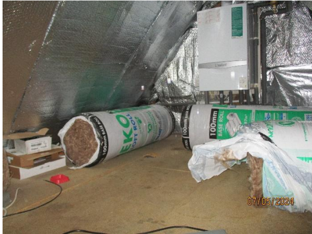
Photo 13: Internal of Void 3.
