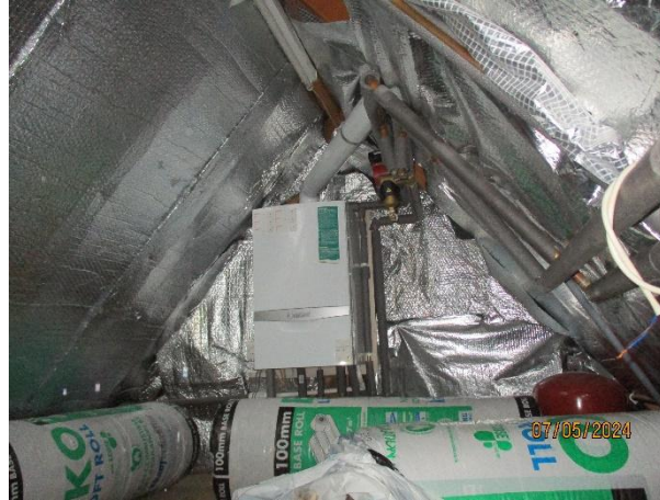
Photo 14: Internal of Void 3.
