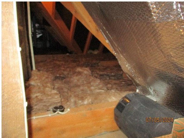
Photo 16: Internal of Void 2, viewing Main Void.
