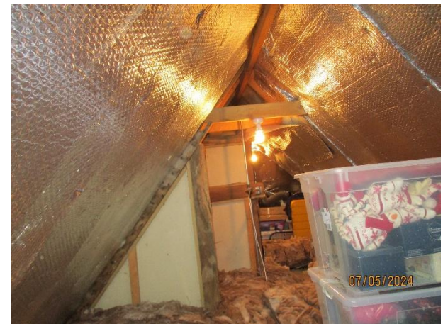
Photo 12: Void 1, viewing Void 2.
