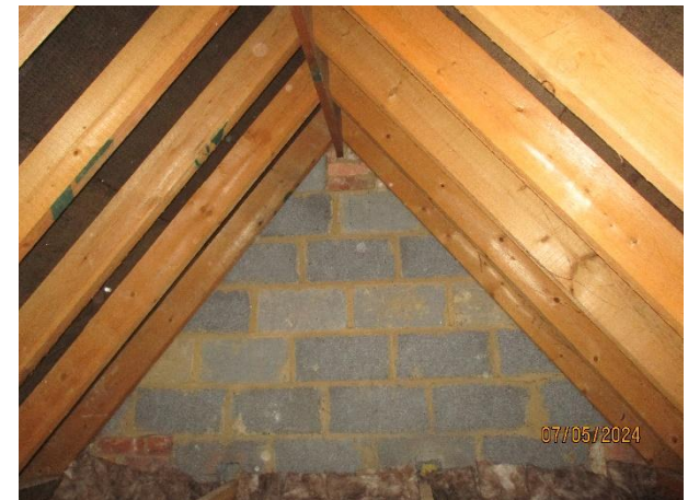
Photo 18: Internal of Main Void.
