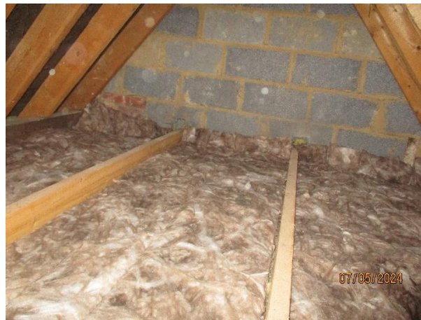
Photo 17: Internal of Main Void.
