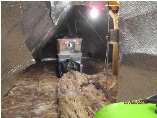
Photo 10: Internal of Void 1.
