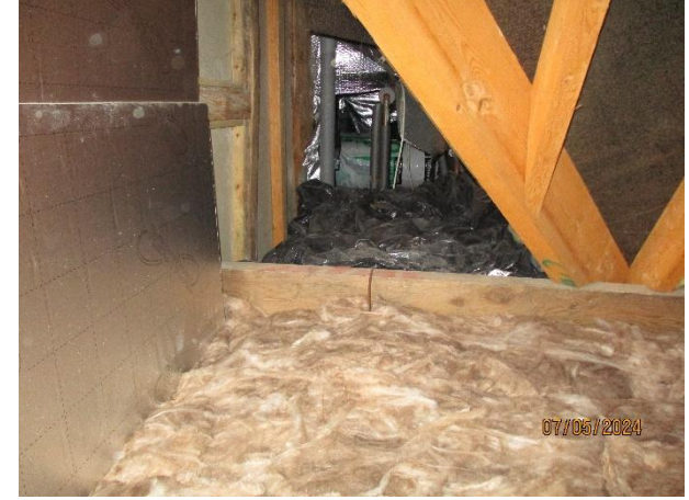
Photo 15: Internal of Main Void, viewing Void 3.
