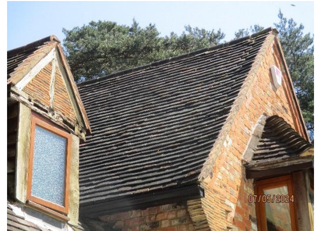
Photo 9: Rear elevation gable end.
